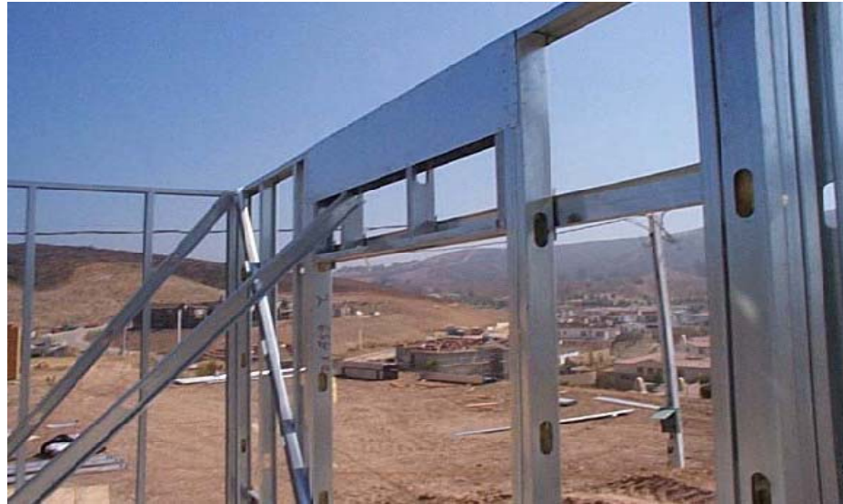
Figure 1.1 Typical Steel L-header (NAHB-RC, 2003)
