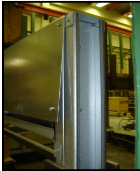
Figure 5.5 Uplift Load Case - Screw failure at Ultimate Load
