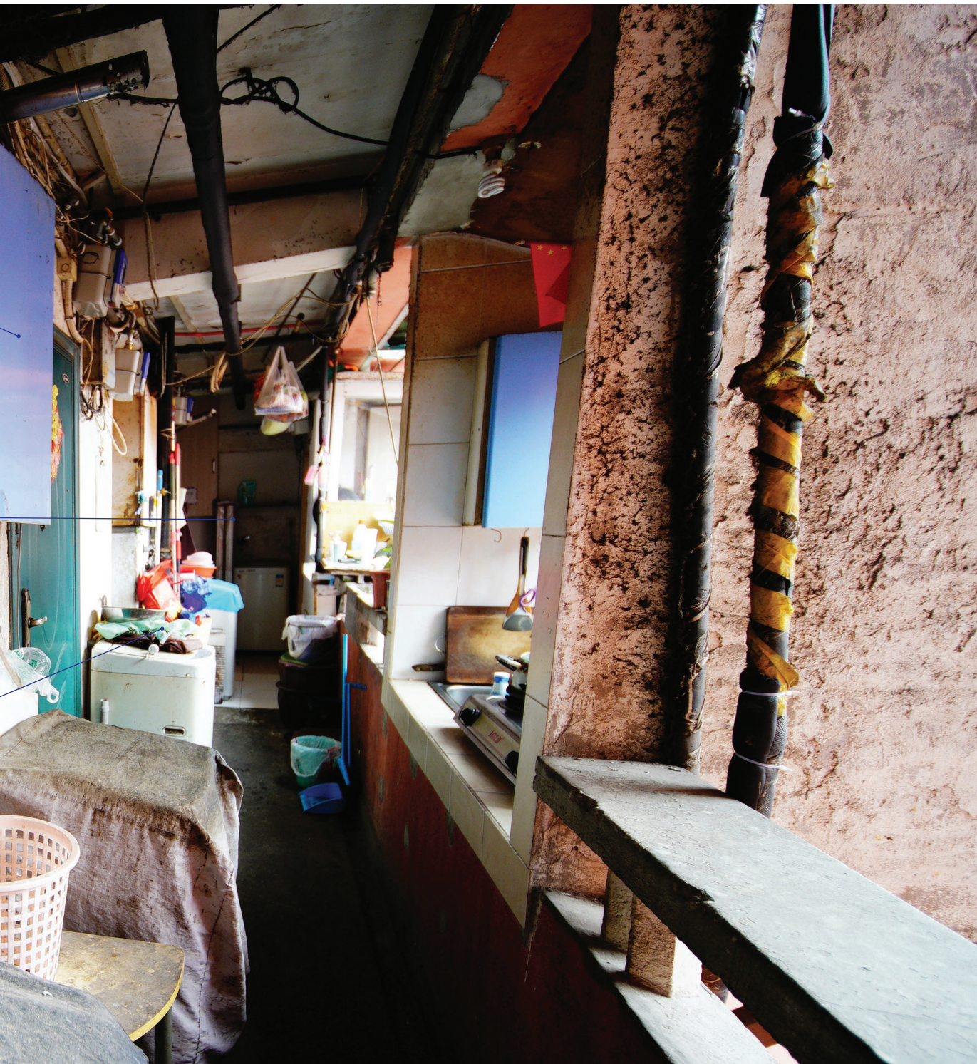
Fig2.29 Photo of Corridor 2
