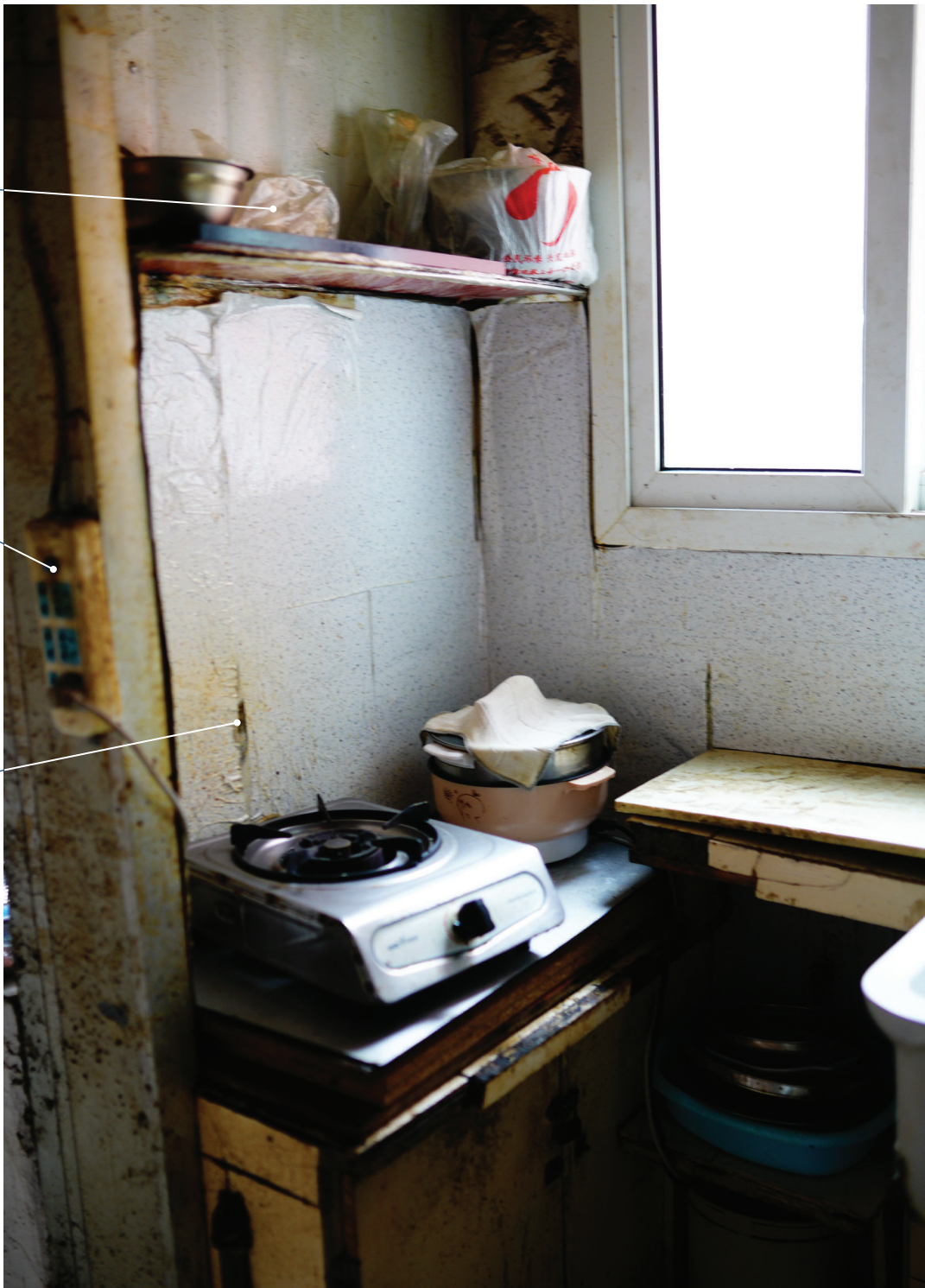
Fig2.24 Photo of Unit 206's Addition
