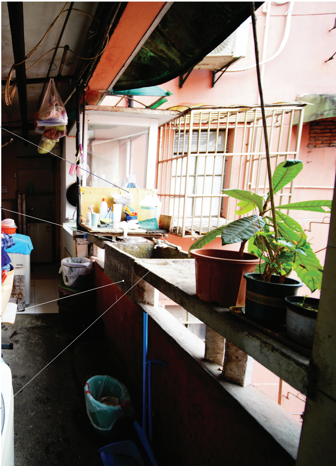
Fig2.32 Photo of Unit 407's Addition
