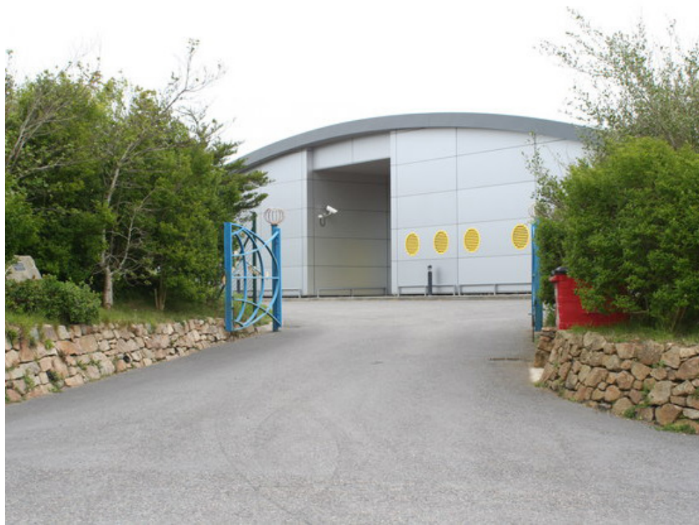
TOP [Fig 1.7]: The new cable landing facility for fibre-optic cables landing at Porthcurno beach at Skewjack Farm. Most cable landing sites are intensely guarded, with restricted access and high security measures. Most stations are further hidden in a facade architecture to make them camouflage into existing urban fabrics.
