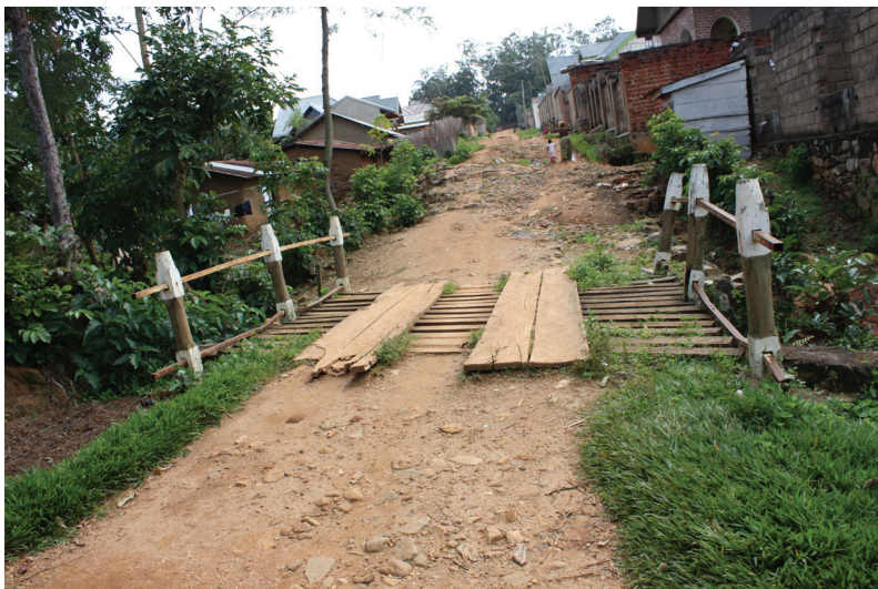
2-40 Enumerators collecting bridge information
