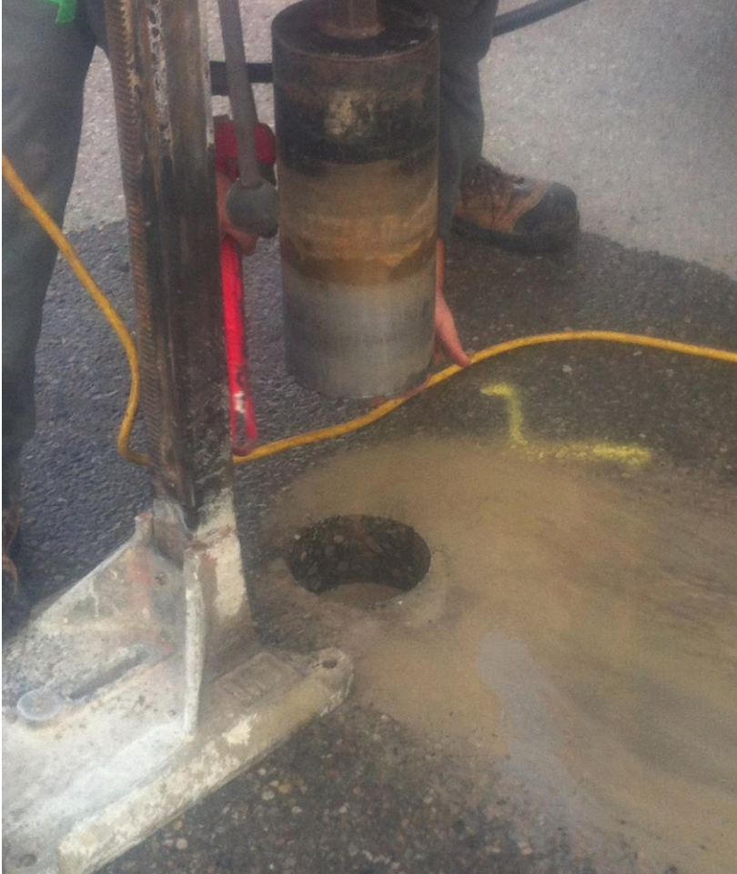
Figure 8.36: Coring of test track in progress
