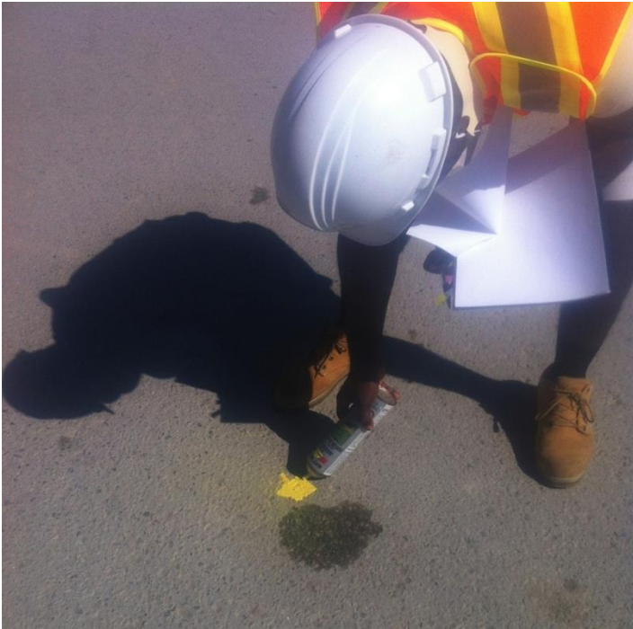
Figure 8.35: Road being marked for coring
