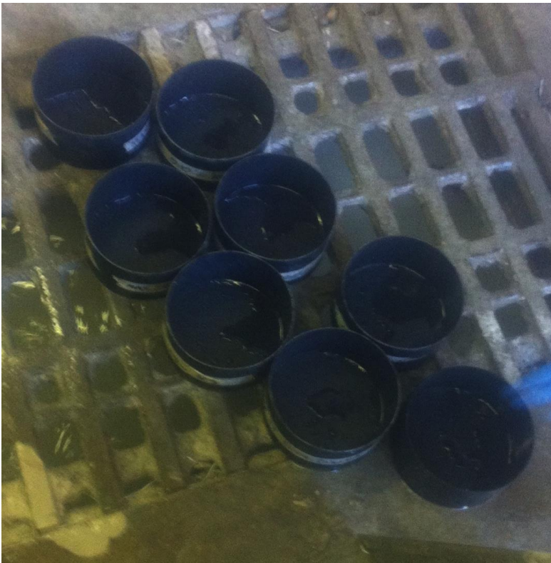
Figure 8.7: Plastic molds washed and are made ready for concrete to be poured
