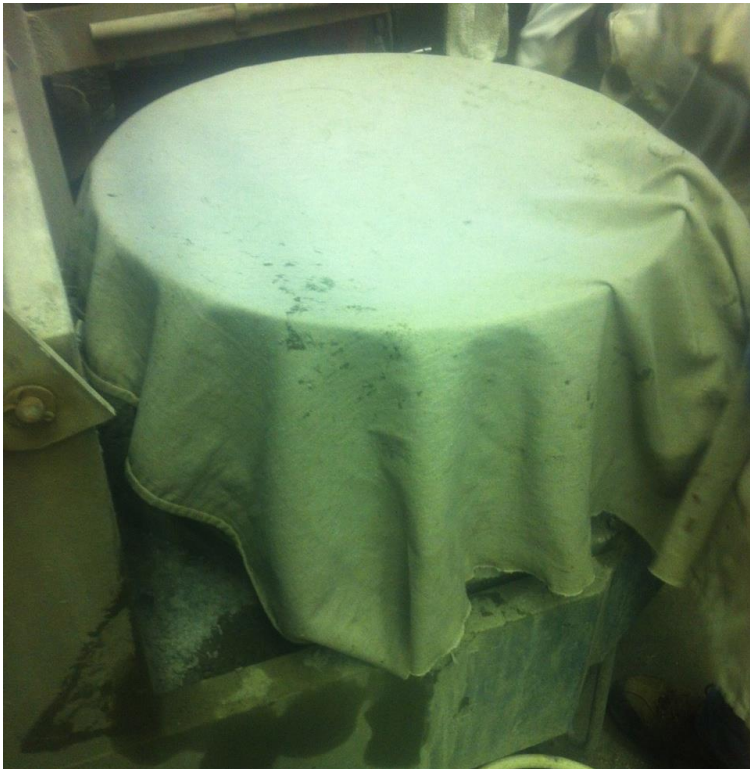
Figure 8.5: Wet burlap placed on concrete to aid hydration process
