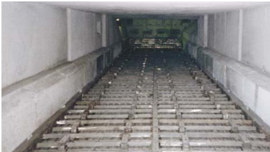
Figure 2-3: Grate clinker cooler [22]
