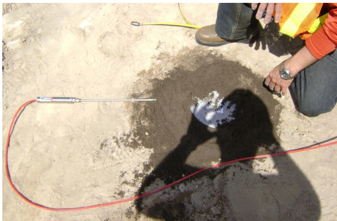
Figure 15 - Earth Pressure Cell Installation
