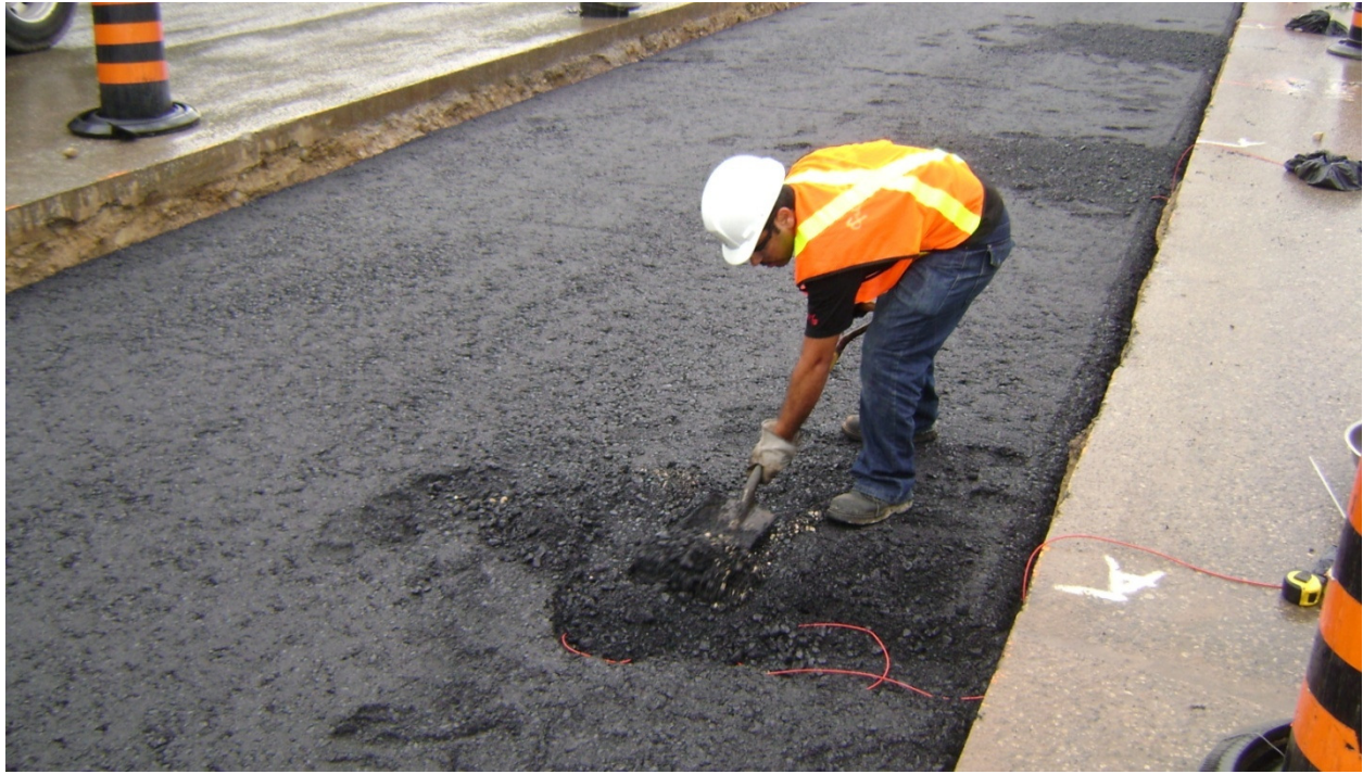
Figure 19 - ASG Installation at Between RBM and SP 25 Layers
