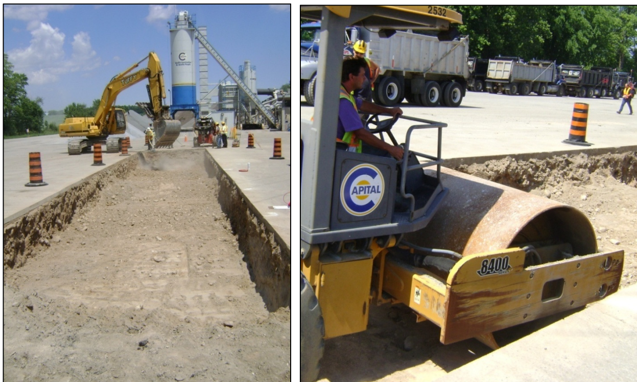
Figure 14 - Preparation of the Subgrade for EPC Installation
