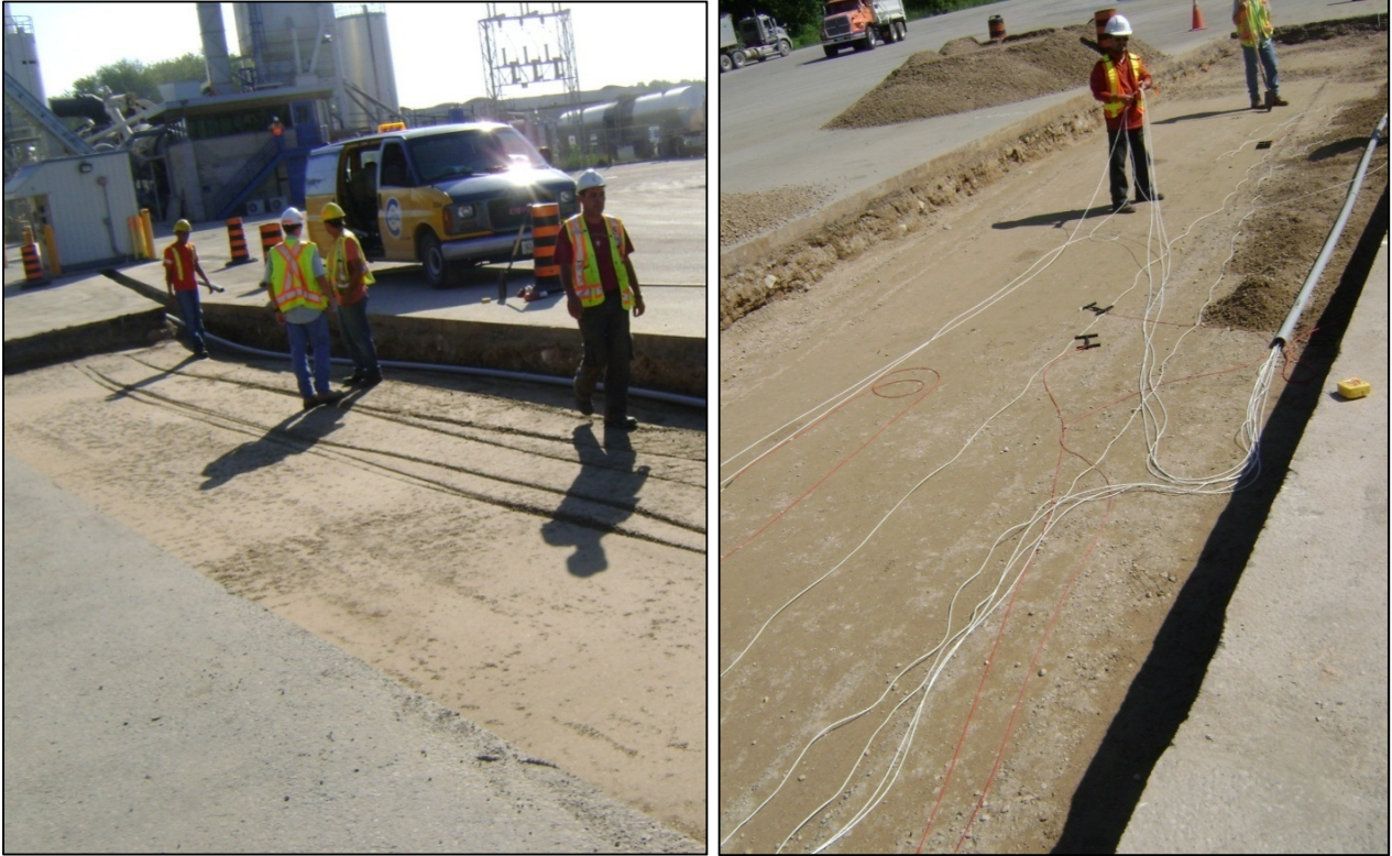
Figure 17 - ASG Installation within Trench Leading to Ticket Room
