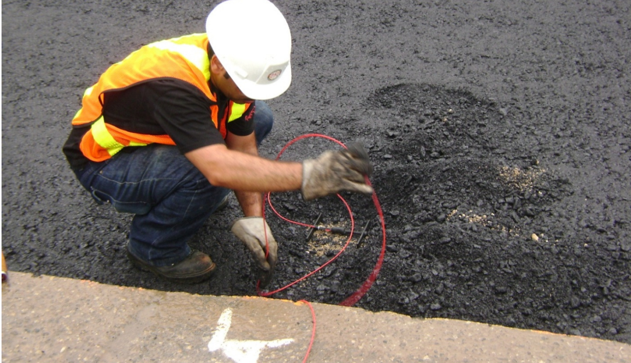
Figure 18 - ASG Installation at Bottom of RBM
