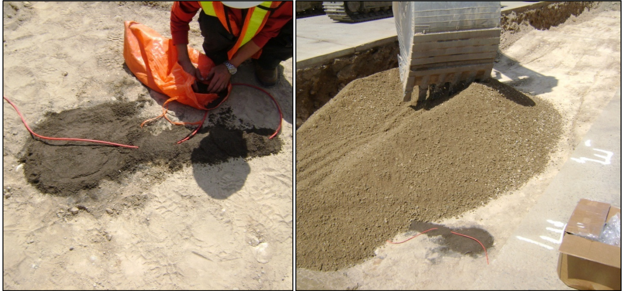
Figure 16 - Earth Pressure Cell Protection During Subbase Construction
