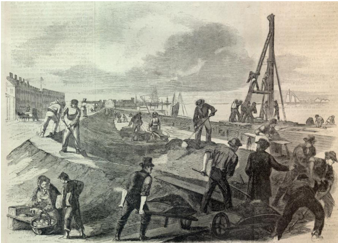
Fig. 2.7. Repairing the levees at New Orleans, at the expense of United States government, sketched by an occasional correspondent, 1863.
