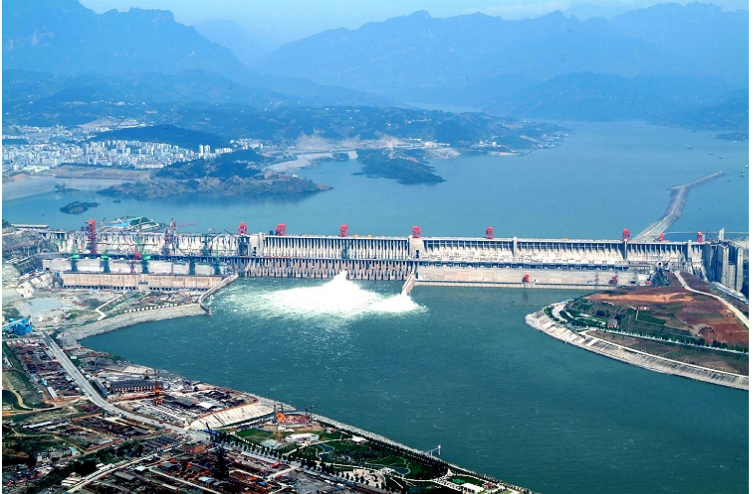
Fig. 2.9. Three Gorges Dam, Yangtze River, China.
