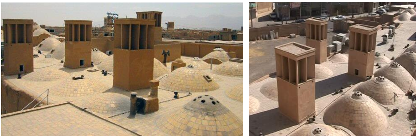
Figure 16. Combination of dome and flat roofs in Yazdi traditional houses, photo by Reine
