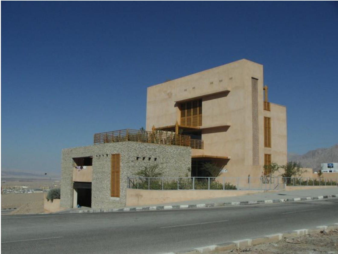
Figure 90. The low energy residence in Aqaba, Jordan
