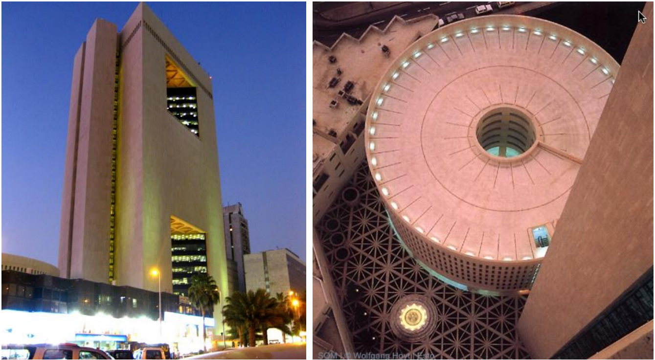
Figure 89. The sky-courtyards are shown in the left picture and the circular parking in the right
