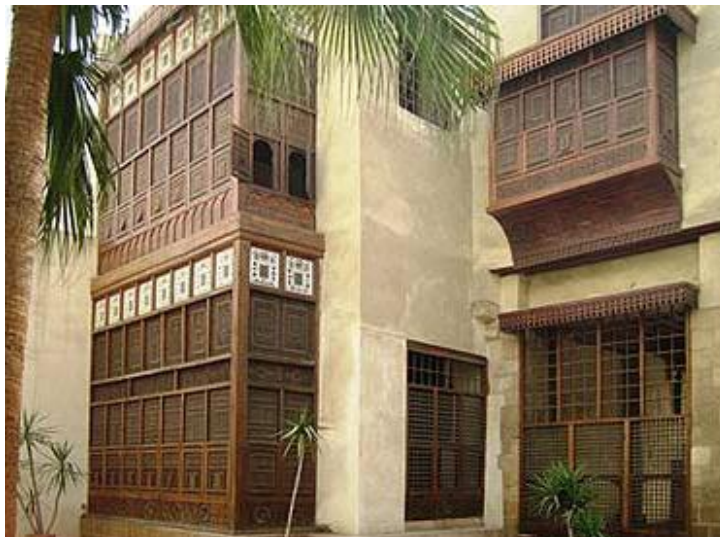
Figure 21. Traditional exterior shading in Cairo, Egypt
