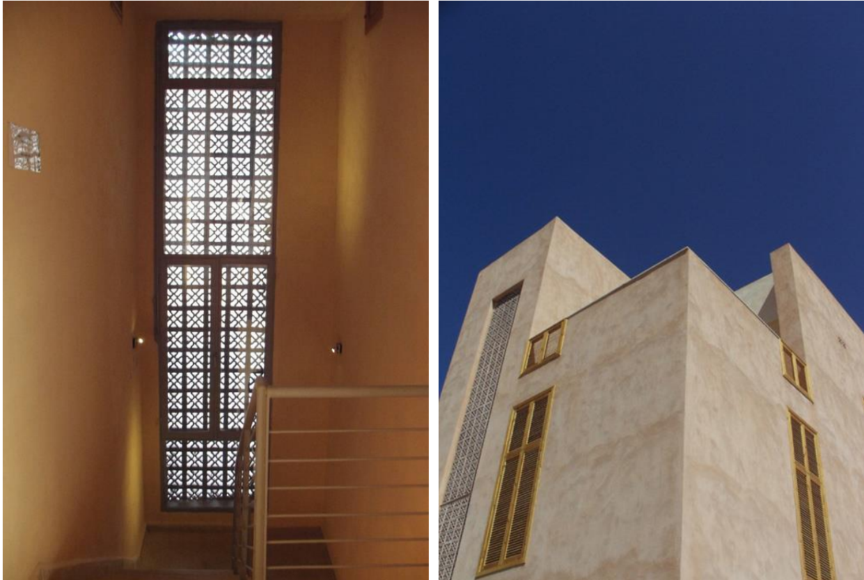
Figure 91. The main staircase is designed to work as a wind tower; view from inside and out
