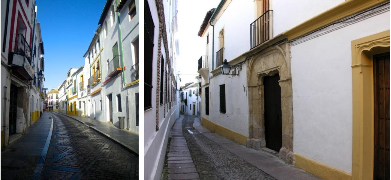
Figure 62. The urban fabric in the historic area
