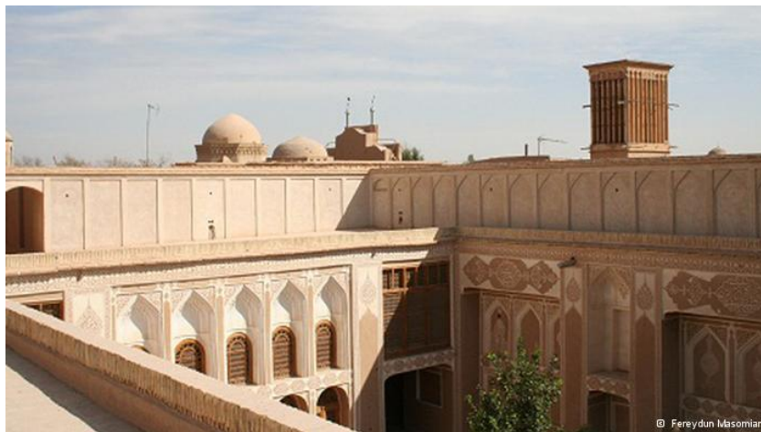
Figure 18. Self-shading in a traditional courtyard house in Yazd, photo by Fereydu Masomian
