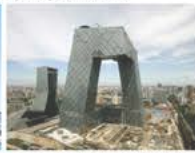
CCTV - Beijing, China
