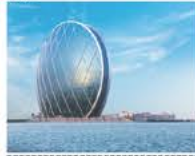
Aldar HQ - Abu Dhabi, UAE
