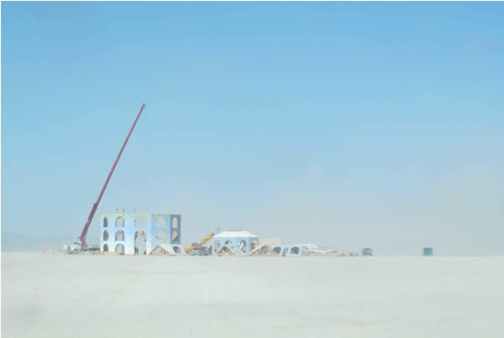
Figure 39 - Man Base Under Construction
