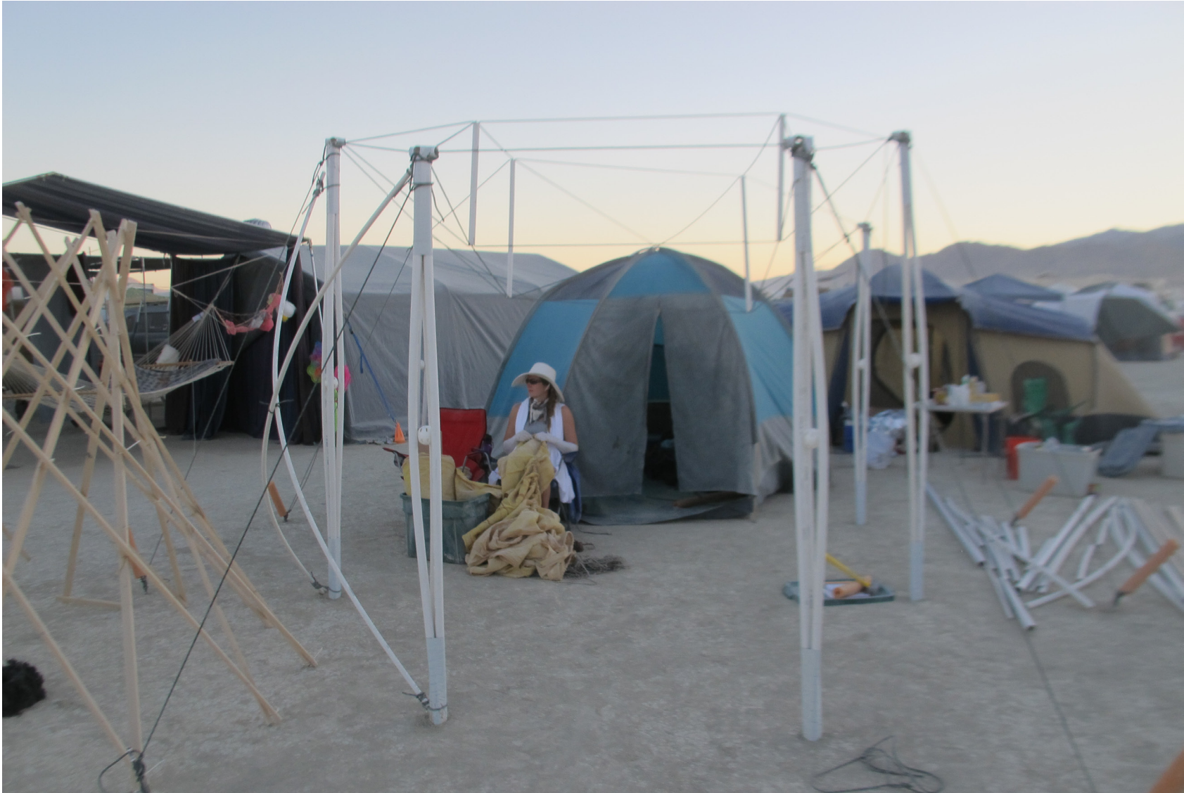
Figure 71 - Constructing the Pearl Palace
