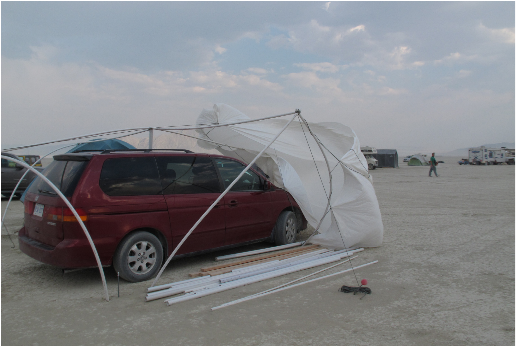
Figure 47 - Shade Structure in a Wind Storm
