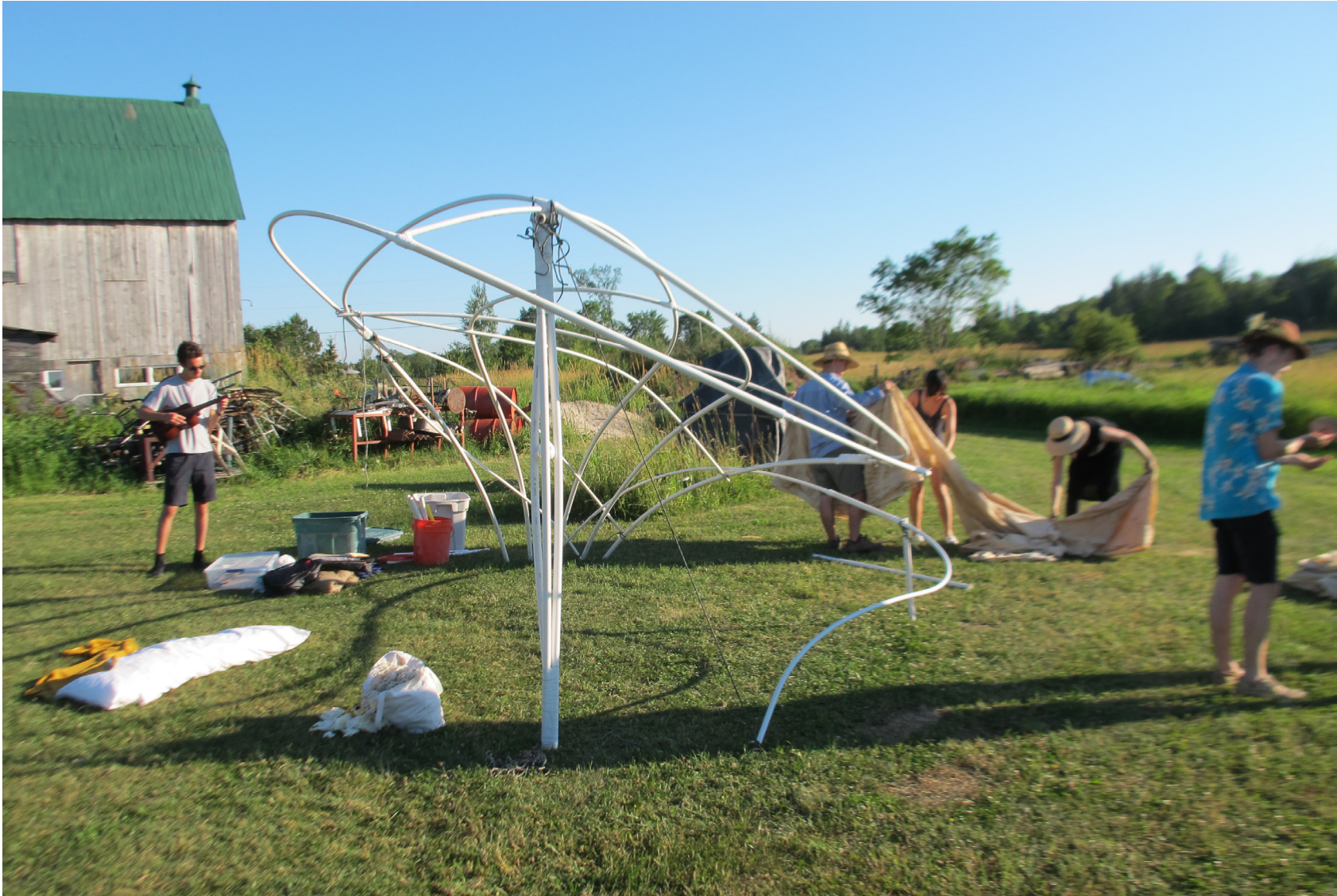
Figure 106 - Pearl Palace Structure
