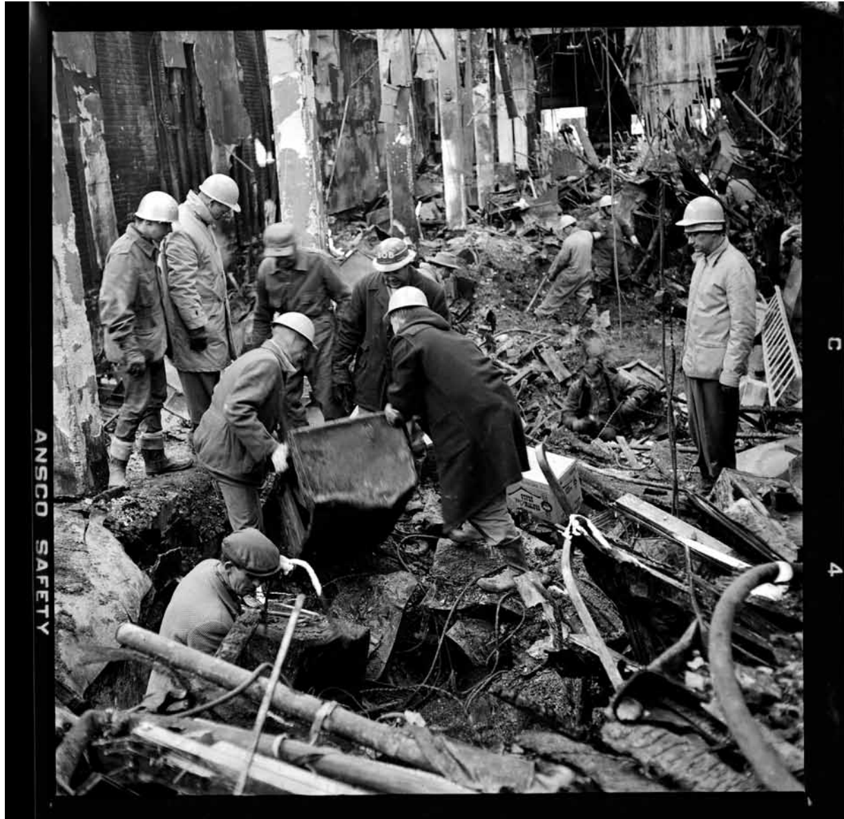
Figure 10.4 - Digging Through the Rubble
