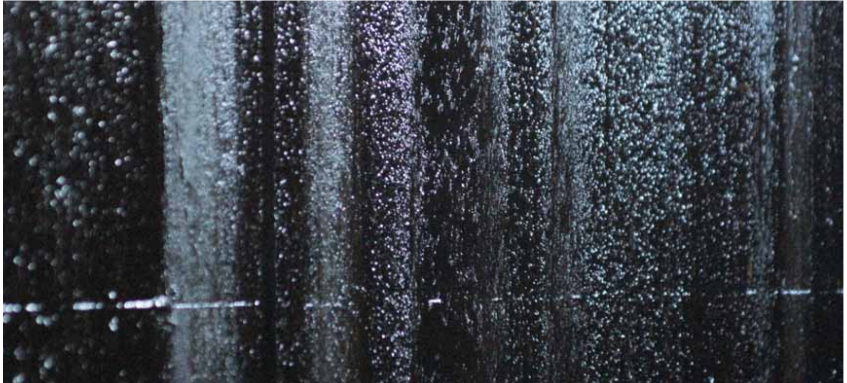
WALLS BLEED BLACK
