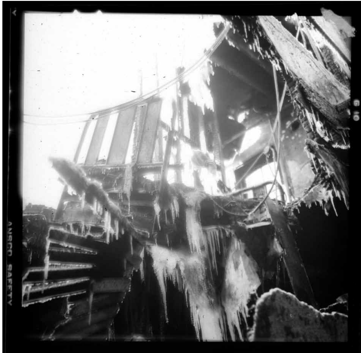
Figure 17.5 - Fire Escape (ii)
