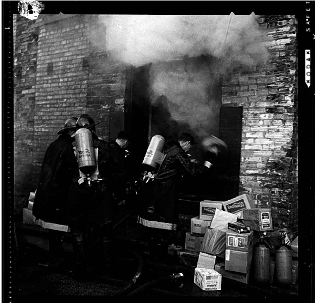
Figure 10.5 - Descending the Furnace
