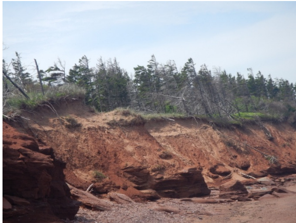
Figure 65: Coastal erosion of bluff system at Cabot Beach Provincial Park, May 2013
