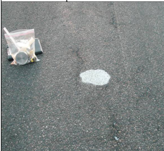
Photograph 3: Sand patch test in area of fatigue cracking on runway
