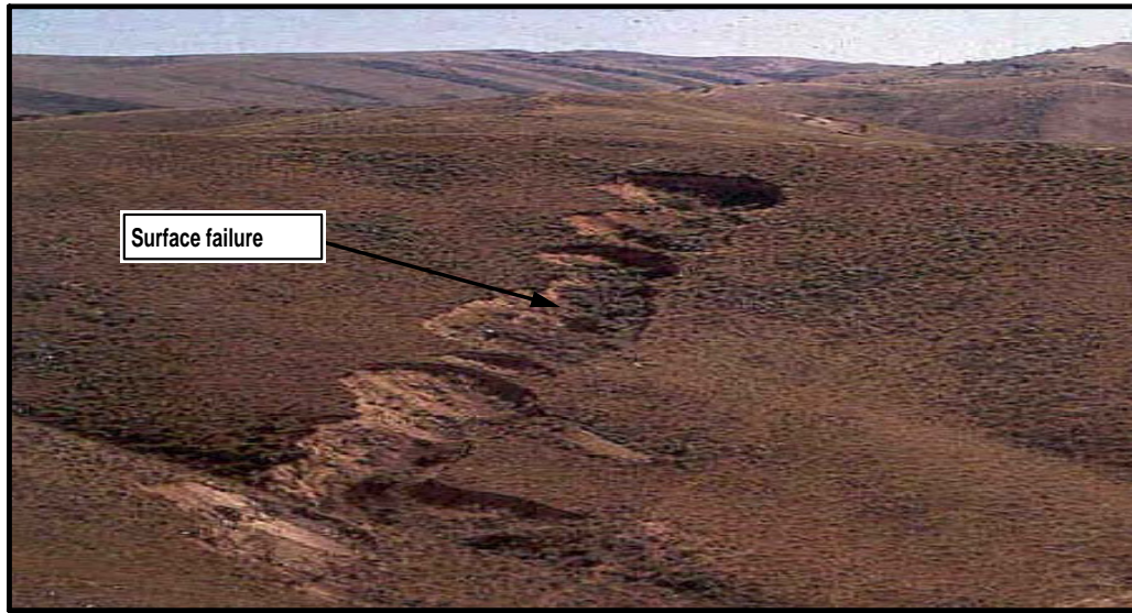
Figure 9-2: Crown pillar failure in Crawford Mountains, Rich County, Utah.
