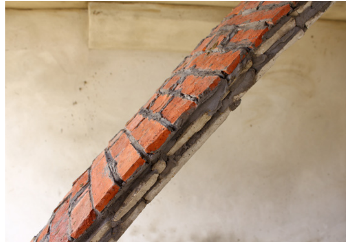
5.2. Overlapping tiles create a Catalan vault.
