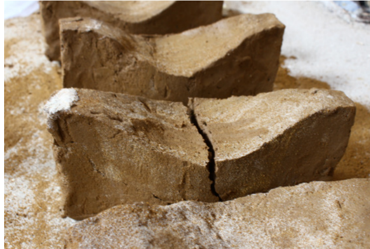
I.17. Brick cracks.
