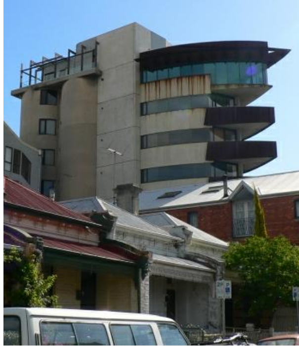
Figure 8: Exterior view of converted apartment shows the addition of balconies. (Kane, 2012)
