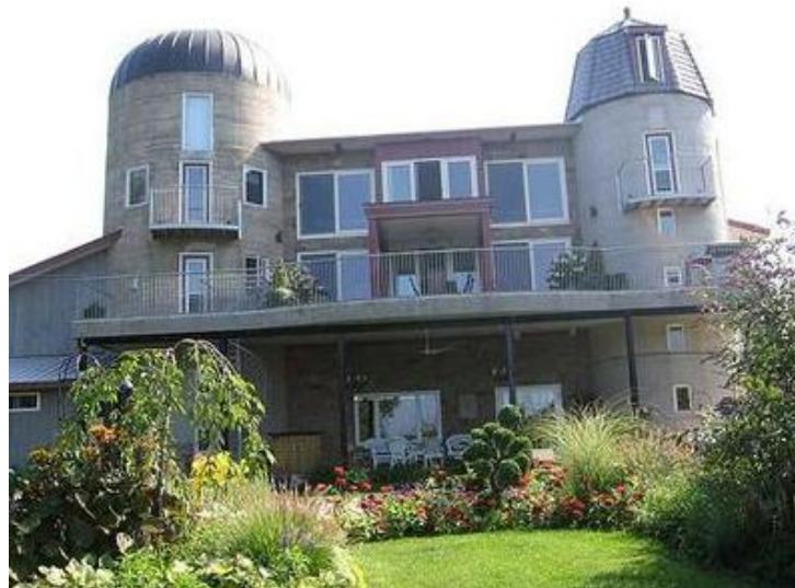
Figure 3: A single family house constructed between two grain elevators in Goderich, Ontario. (Kearney, 2010)
