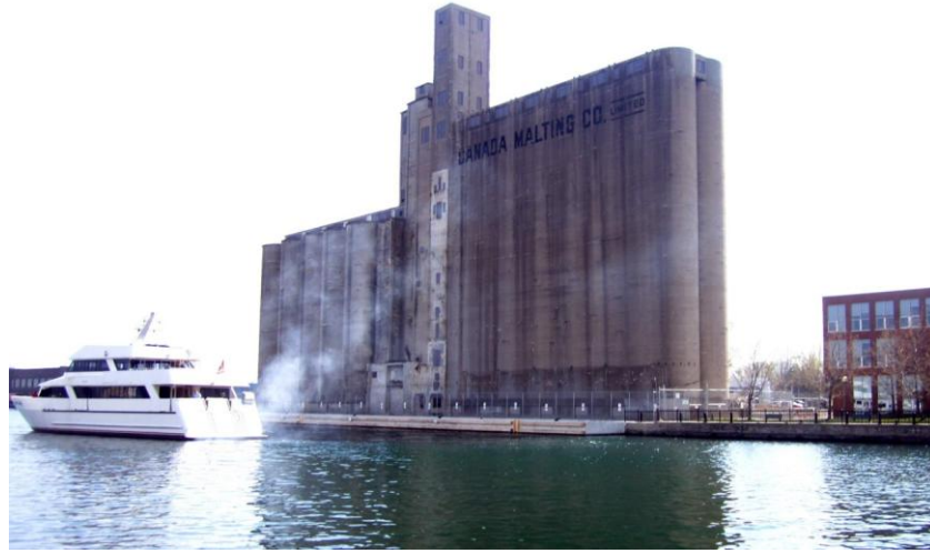
Figure 19: Photo of current state of the Canada Malting Silos (Kevill 2012)
