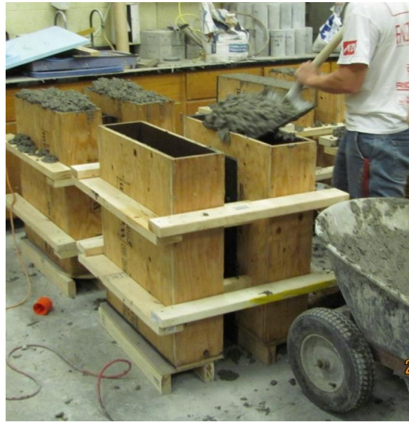
Figure 4-12: Vertical Casting of Concrete Slabs for Control and Shear Lug Specimens
