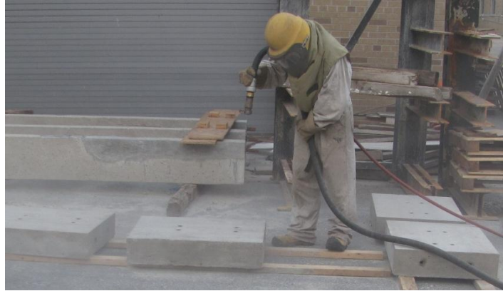
Figure 4-15: Sandblasting of Concrete Slabs
