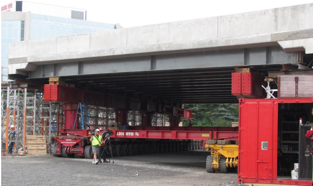
Figure 2-1: Self-Propelled Modular Transporters underneath a Bridge Superstructure
