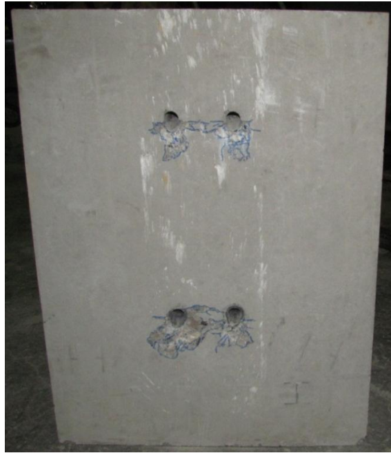
Figure 5-18: Concrete Crushing under the Bolt Holes on Specimen FE1 L-53
