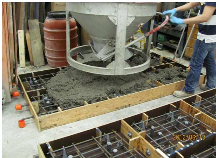
Figure 4-13: Horizontal Casting of Concrete Slabs for Remaining Specimens
