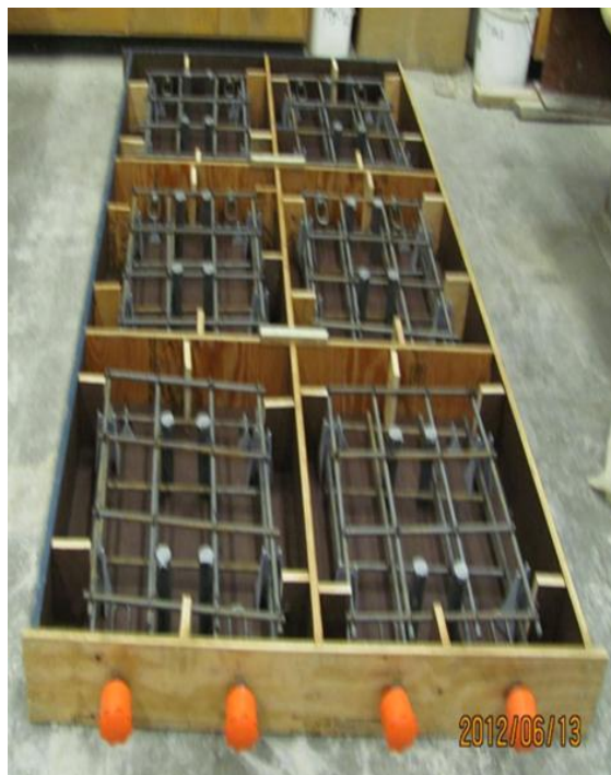
Figure 4-10: Forms for Horizontal Casting of Concrete Slabs
