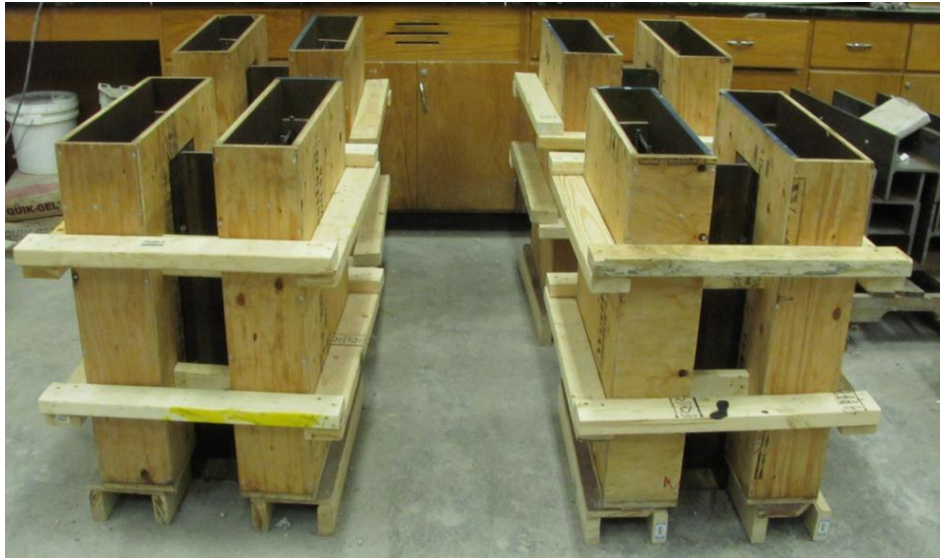
Figure 4-9: Forms for Vertical Casting of Concrete Slabs
