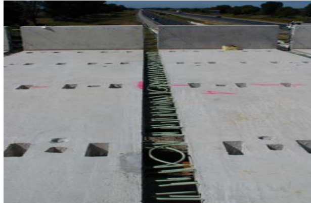
Figure 2-3: Precast Concrete Deck Panels with Grout Pockets [Lam and Tharmabala 2011]
