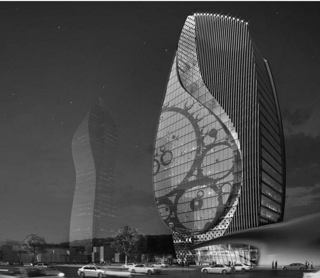
Fig 4.62 Azersu Tower by Heerim Architects & Planners Co. Ltd. Groundbreaking 2012, expected to complete in 2014, 20 Floors, Area 31860 m 2
