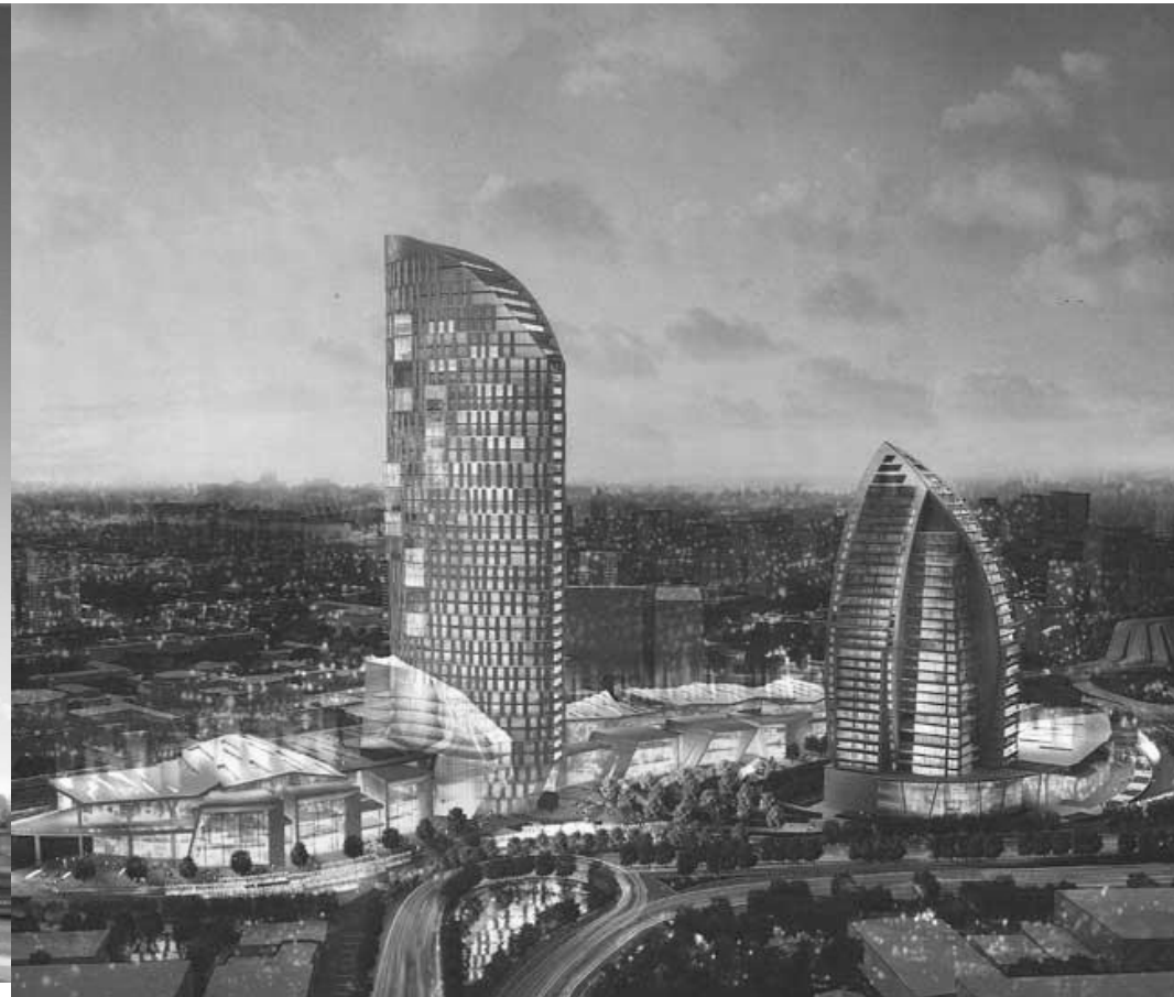
Fig 4.65 Trump Tower by ZQAN Construction 33 storey tower, 130 m, mixed used, expected to complete in 2013
