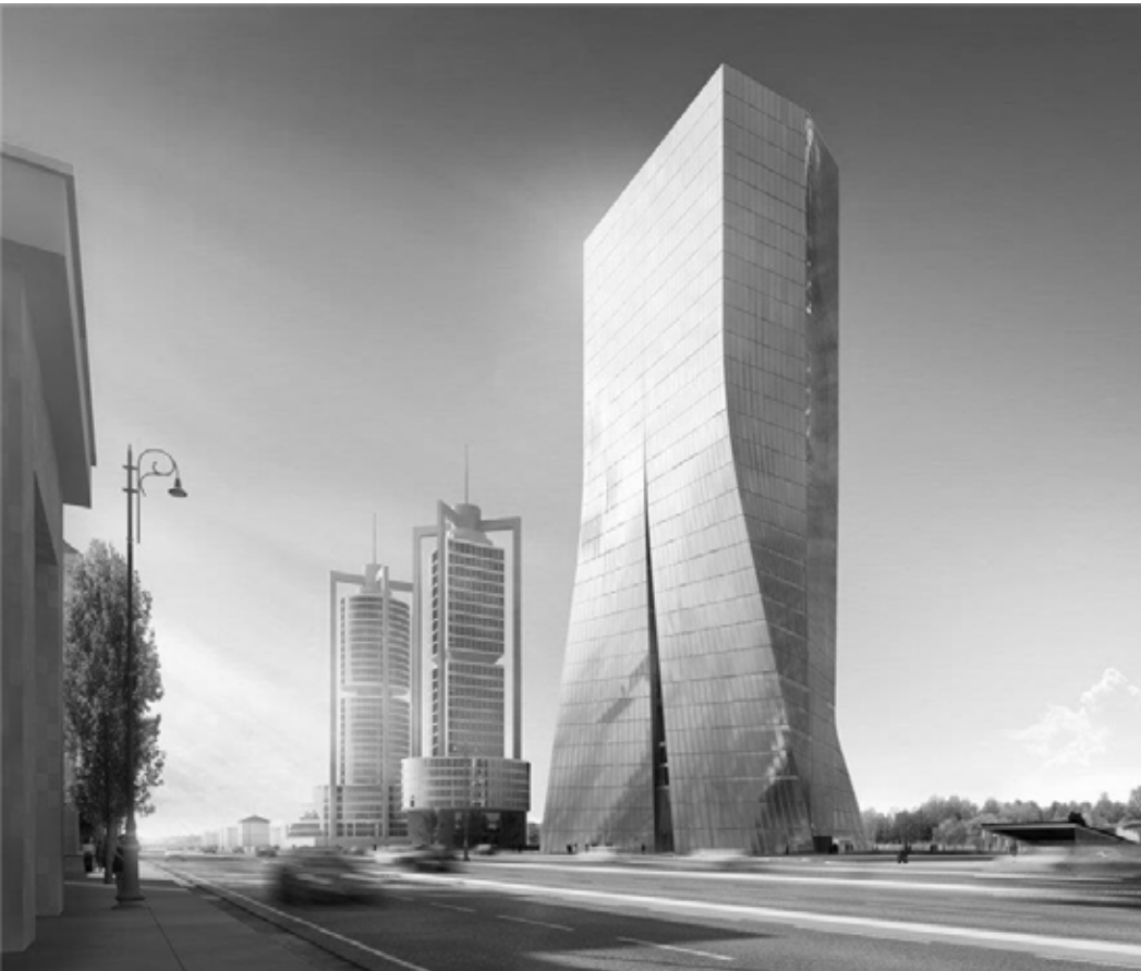
Fig 4.64 Central Bank Of Azerbaijan by Coop himmelblau Architecture Expected to complete in 2015, total area 359 m 2
