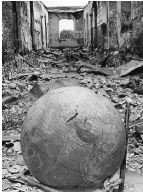
Fig 3.17 Destroyed Agdam high school.
