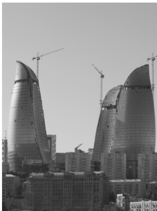
Fig 2.4 Construction boom, Baku, Azerbaijan.
