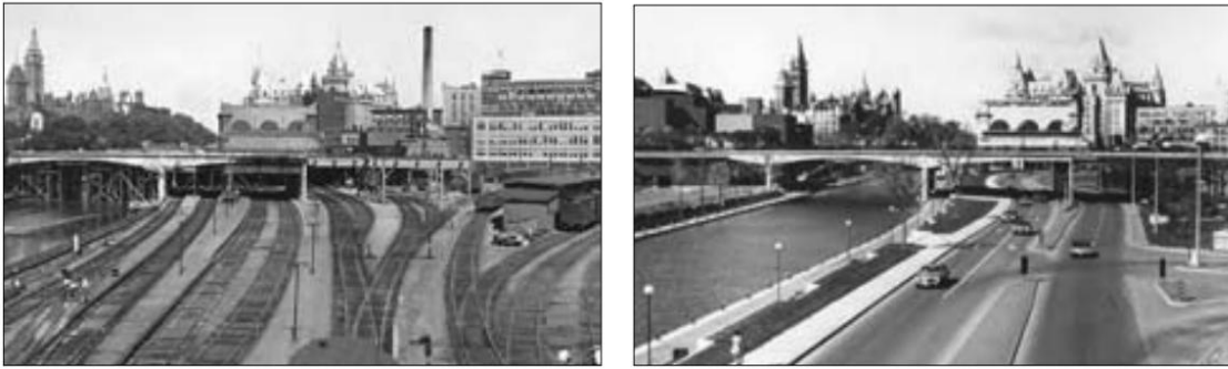
Figure 4.3: Undated photos of the downtown core prior and post rail removal (NCC, 1999)
