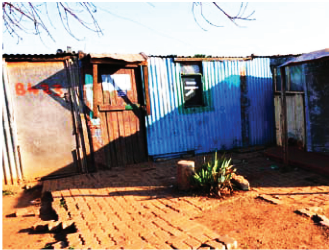
Figure 3.3 Neatly kept shack exterior
