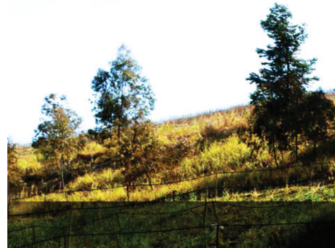
Figure 3.22 Rehabilitation of slope at tailings storage facility
