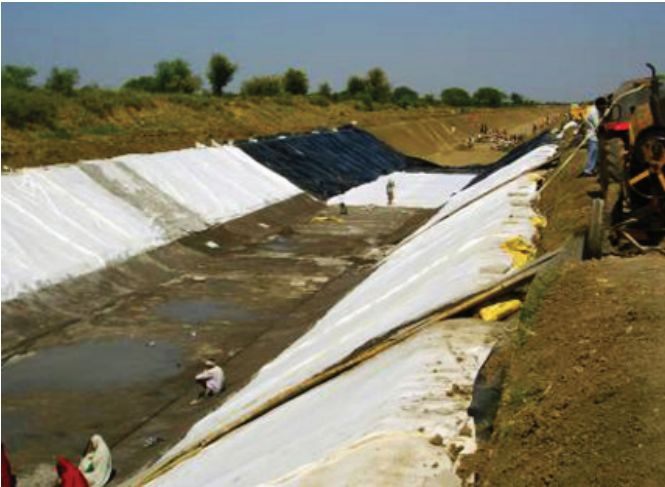
Figure 3.23 An example of a Water Canal during Construction
