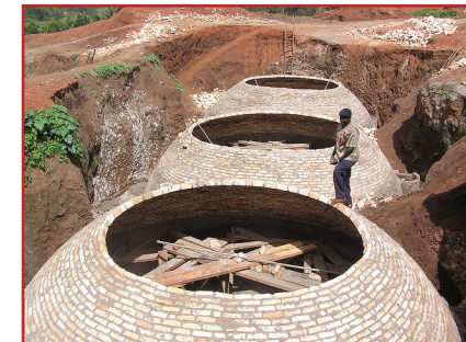
Biogas digester during construction.
