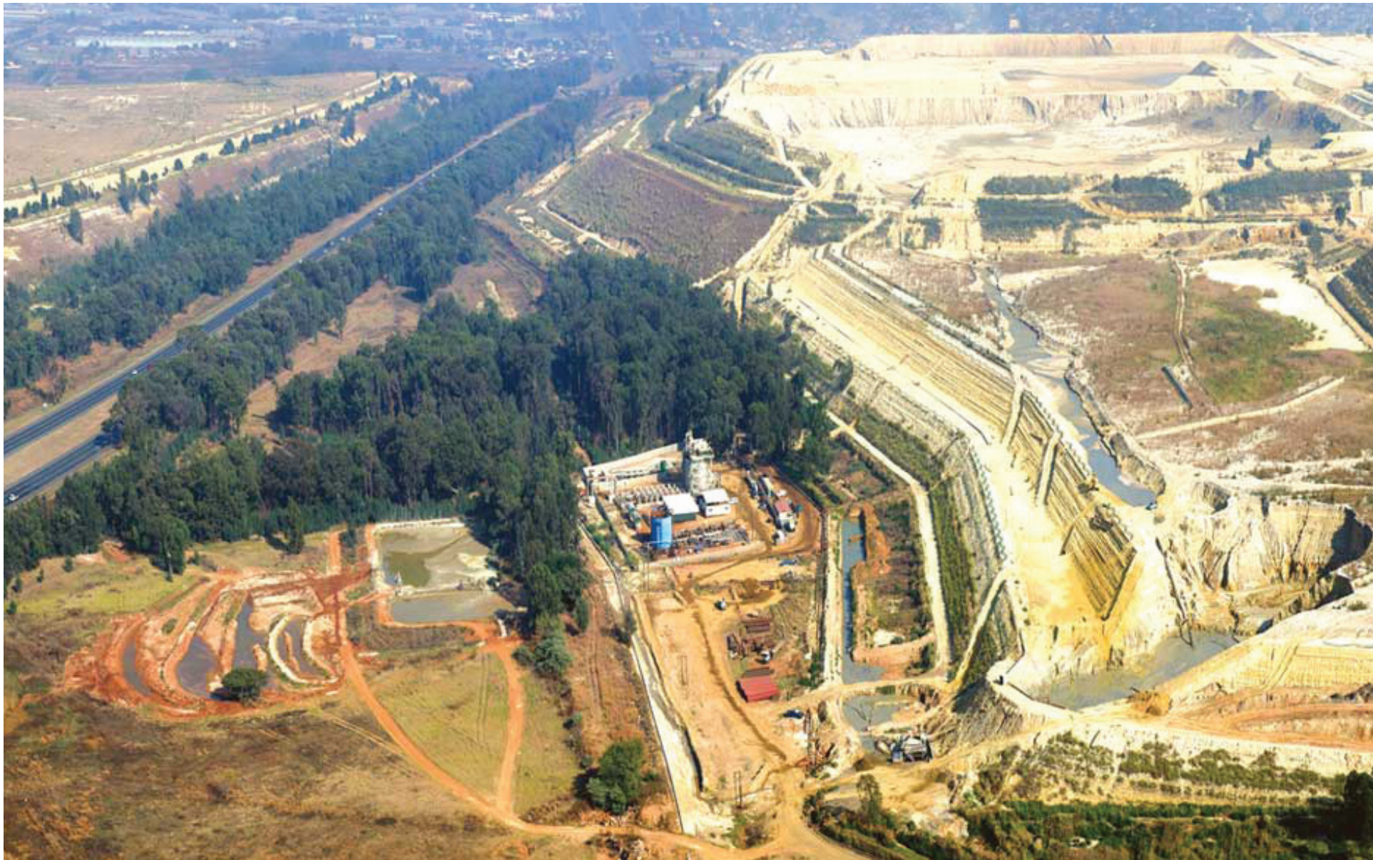
Figure 3.8 An areal view of a tailings storage facility that is undergoing remediation. The slopes have been profiled, a top layer applied and vegetation is starting to grow.
