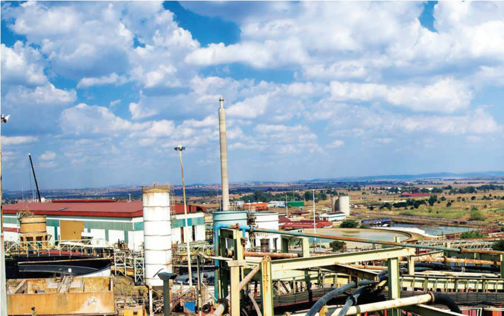
Figure 3.10 Gold mining infrastructure at a plant near the site study area. The design proposes the re-use of this infrastructure to construct new building technologies.
