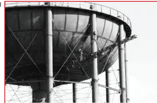
An example of how water towers may be constructed with the existing mining infrastructure.
