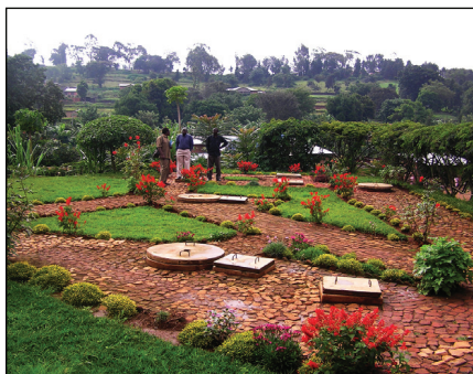
Figure 3.29 Garden above biogas digester
