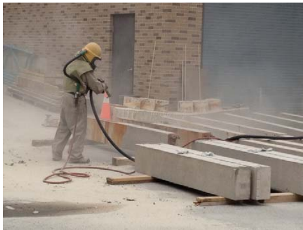
Figure 3.8: Surface sandblasting
