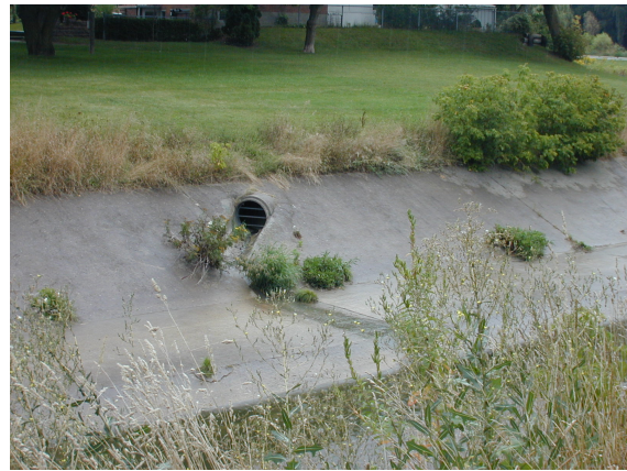
(b) Concrete channel with storm drain
