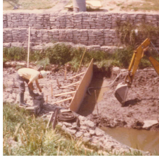
(b) Spring 1975 (control installation)
