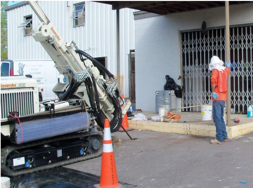
Figure G.1. Angled drilling under the meter shop.
