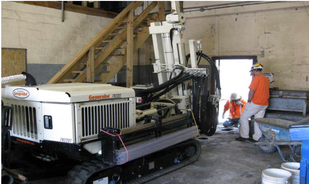
Figure G.2. Drilling inside operations building.
