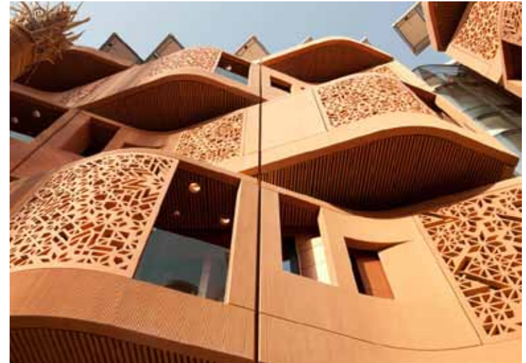
Figure 3.28 Glass-reinforced concrete mashrabiya screens shield the residential buildings' balconies
