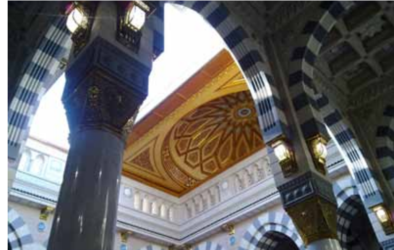
Figure 1.25 An operable dome One of the 27 moving domes installed in the mosque
