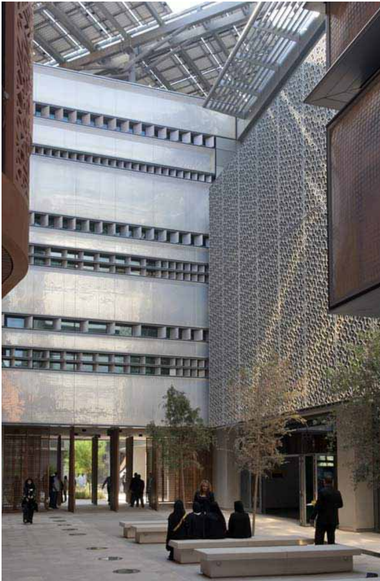
Figure 3.30 Photovoltaic panels project from the roofs over the edges of the courtyards and streets, providing shade and energy generation
