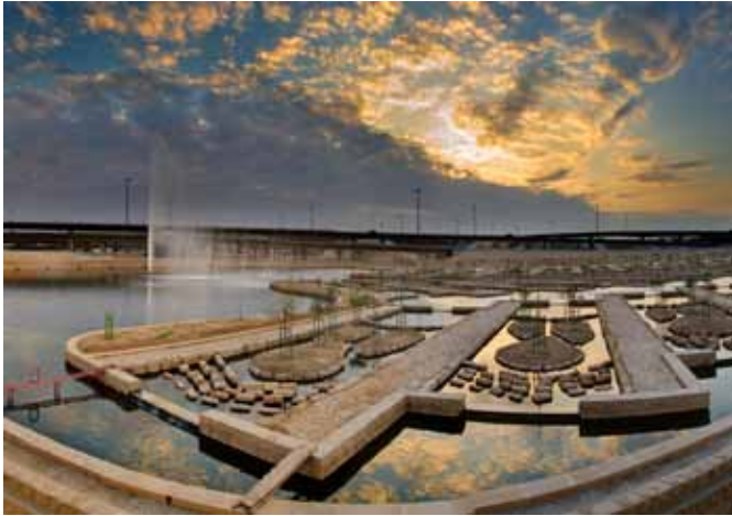
Figure 3.18 Wastewater treatment plant, Wadi Hanifah, Saudi Arabia
