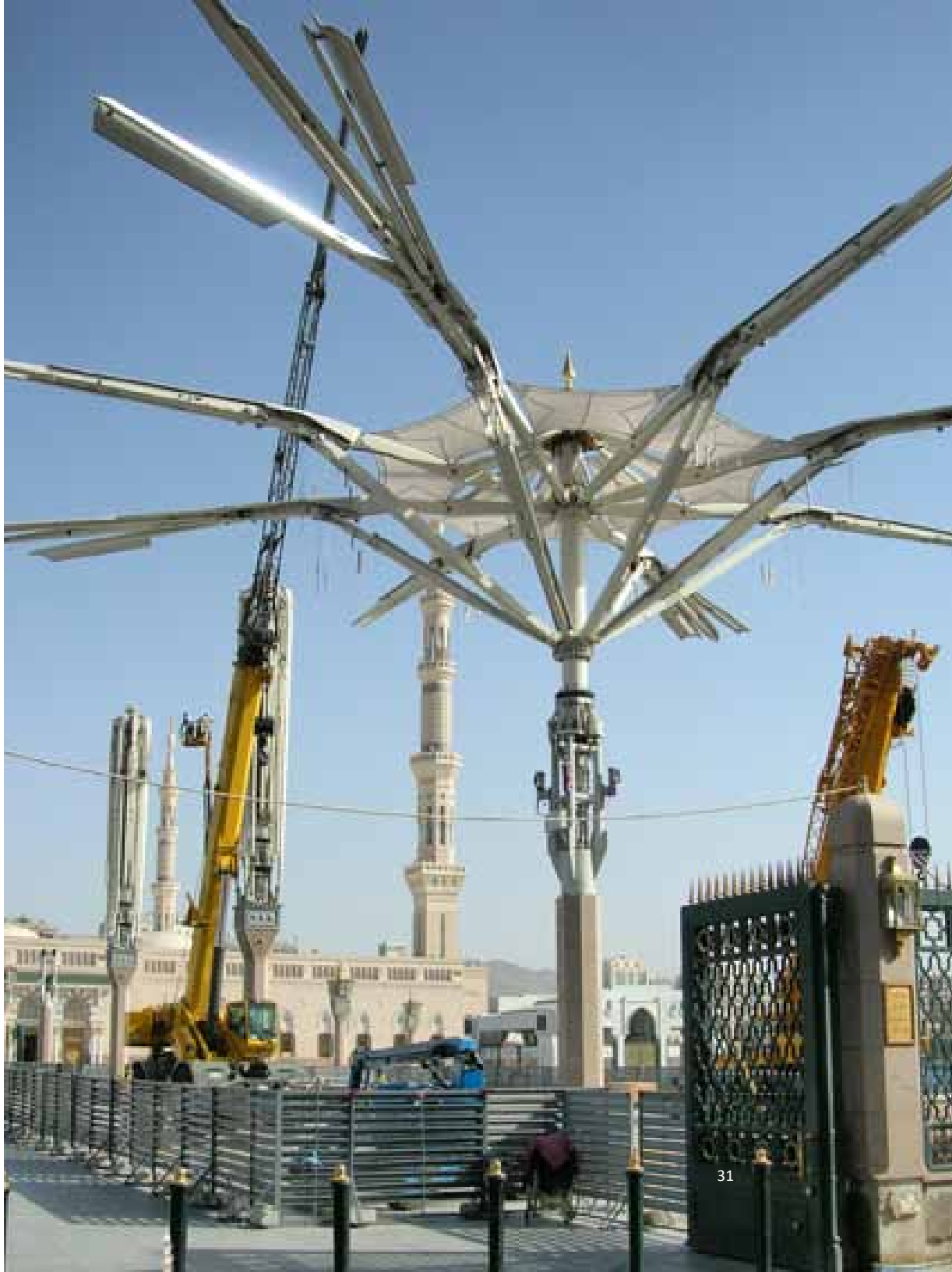
Figure 1.29 The structural arms of the umbrella
