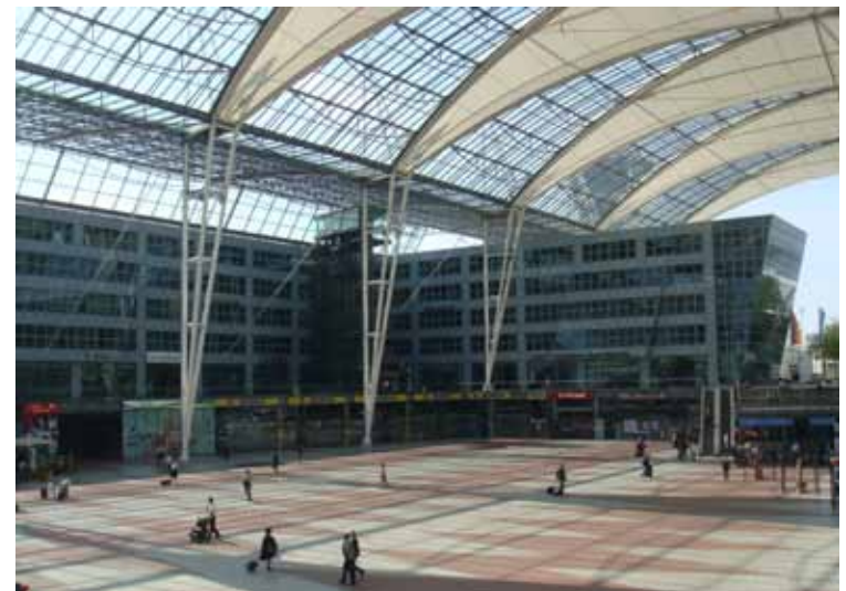
Figure 3.41 Interior view showing the scale of the canopy, courtesy of Andrea Nagy
