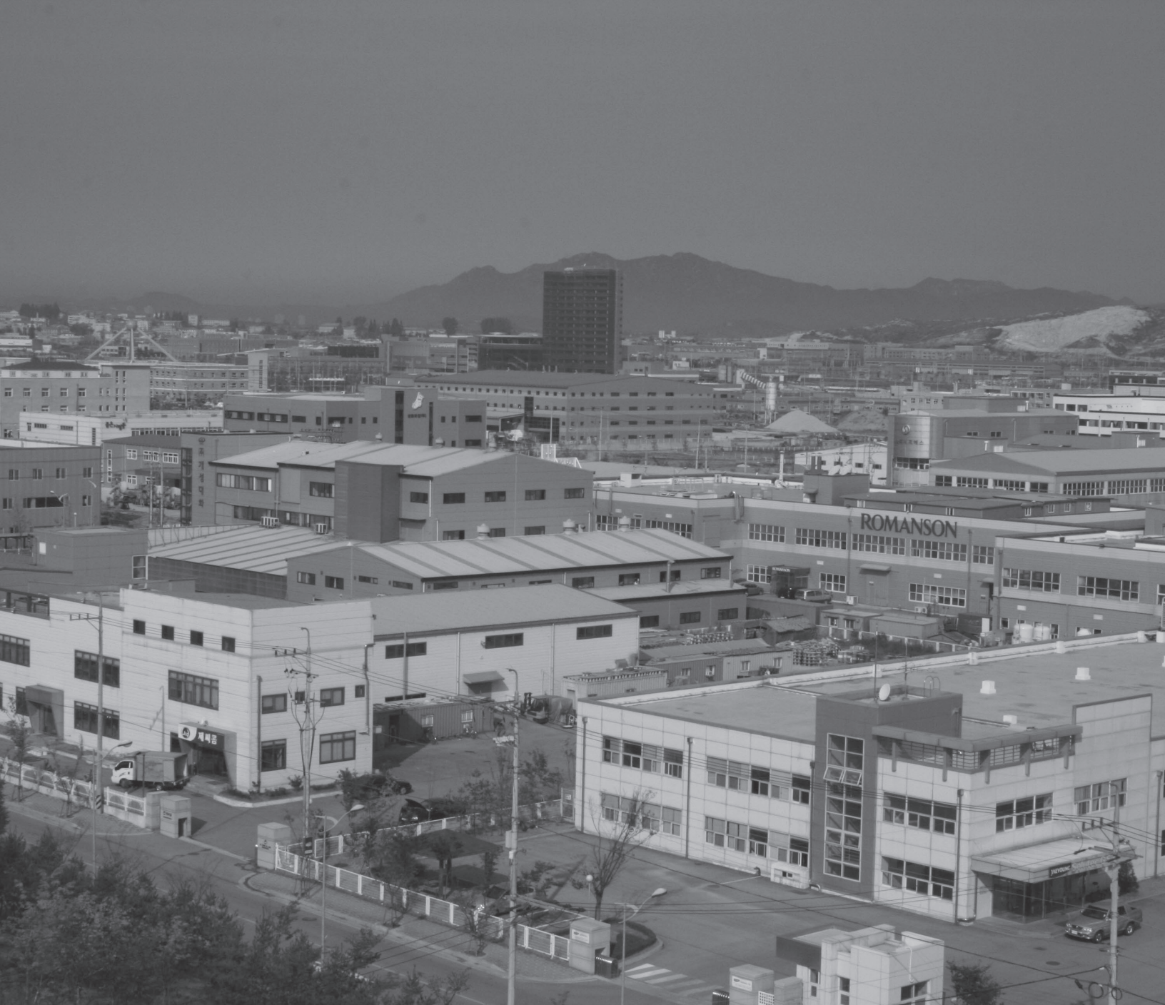
fig. 2.2 View of Gaecheon Industrial Complex
