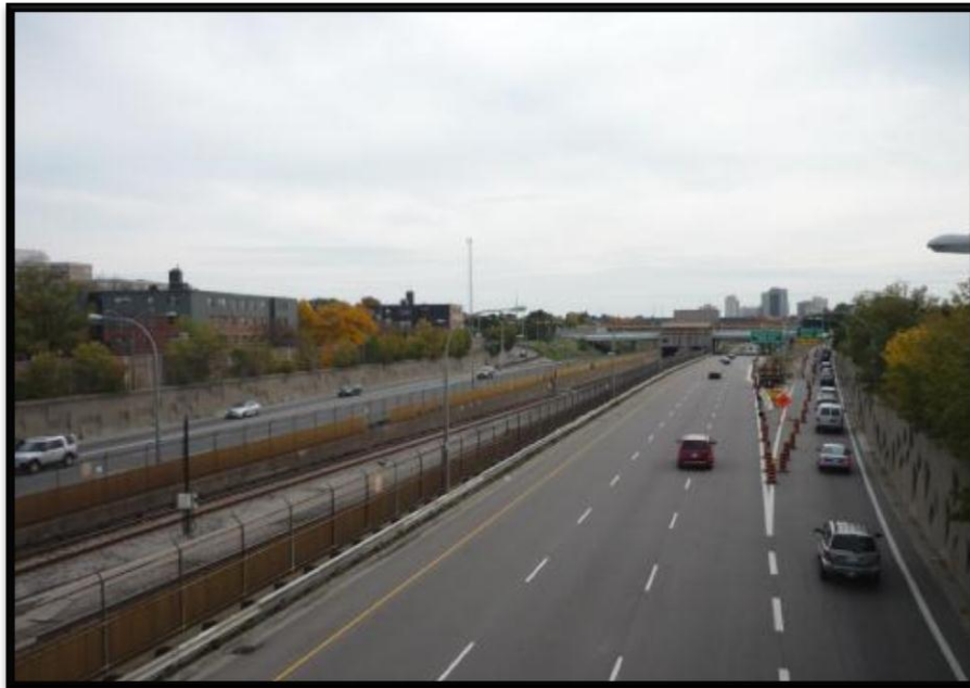
Figure E4 - 2012 – Spadina expressway looking south to Lawrence Ave.
