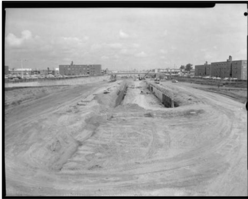
Figure E3 - 1963 – Spadina Expressway looking north at Lawrence Ave.
