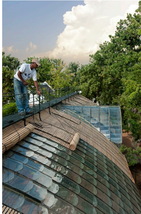
Figure 90: Energy Efficient Cooling (Babylonstoren.com, 2012)
