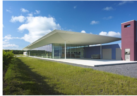
Figure 42: One of the Terraces and the Iconic Roof (Southbrook.com, 2012)
