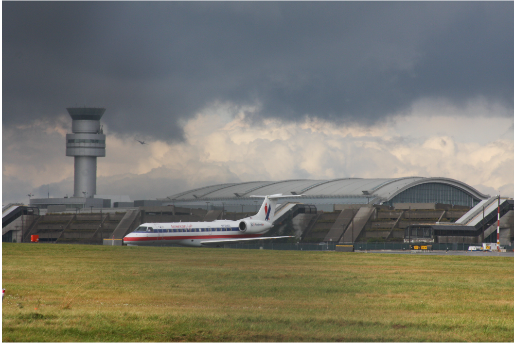
Figure 7.5: Toronto Pearson International Airport Terminal 1 Apron Tower
