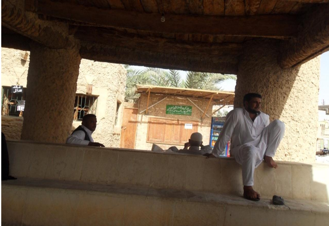
Figure 4.1.2: The bus station (built from traditional materials including palm trunk)
