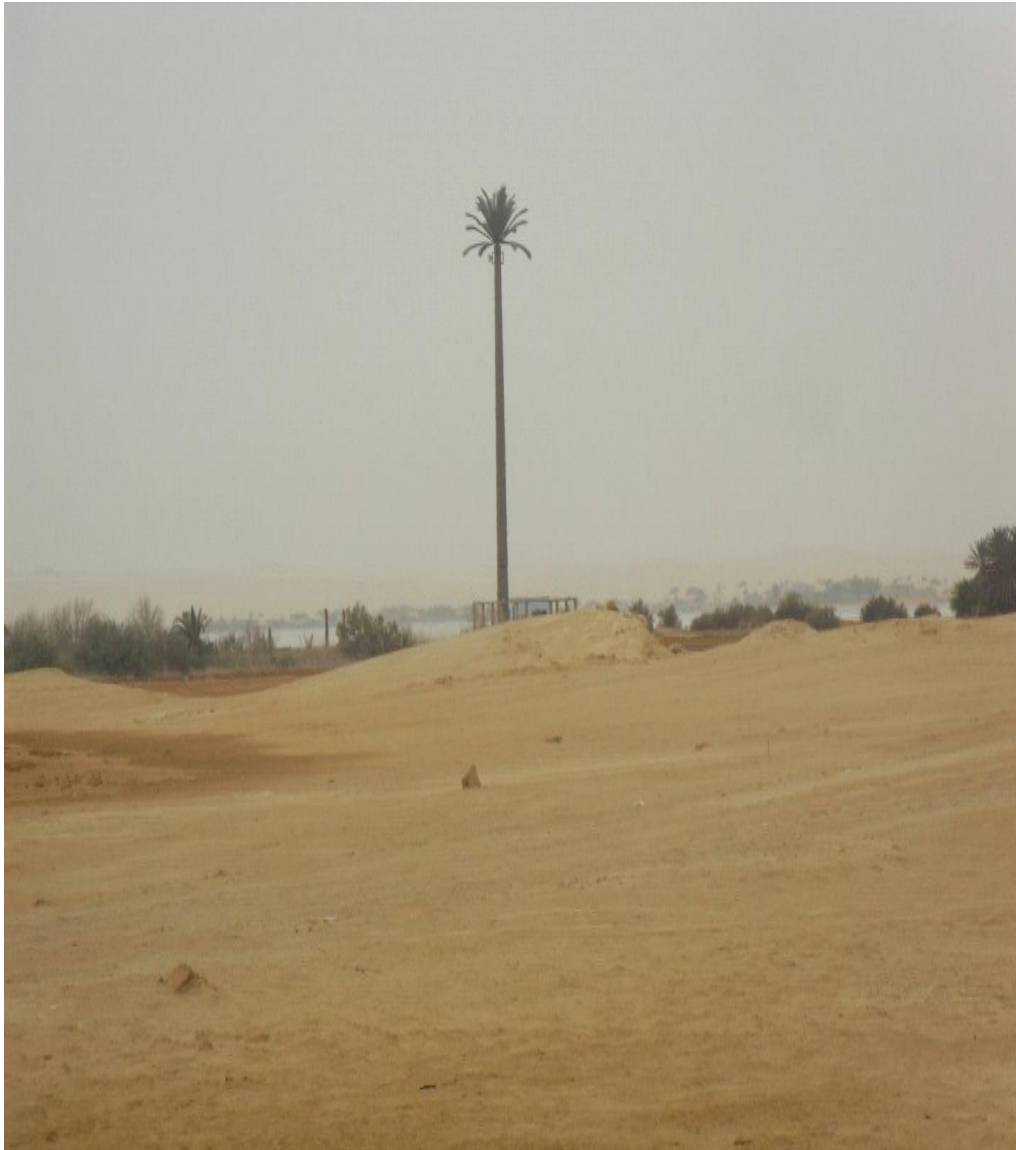
Figure 4.1.5: Part of the Siwan desert on the way to the Adrere Amellal hotel and Taghaghien Island hotel. This artificial palm tree is the focus of a cell phone network which covers the whole oasis
