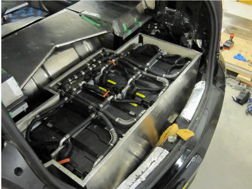
Figure 3.5: 250 V Battery Pack[53]
