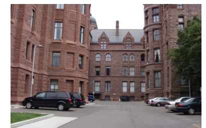
Fig 3.9 North Block Parking Lot
