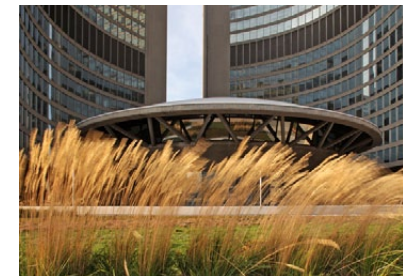
Fig 2.27: New Green Roof Garden on Podium
