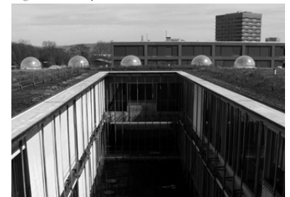
Fig 4.29 Rooftop Garden in Rehab Centre, Basel
