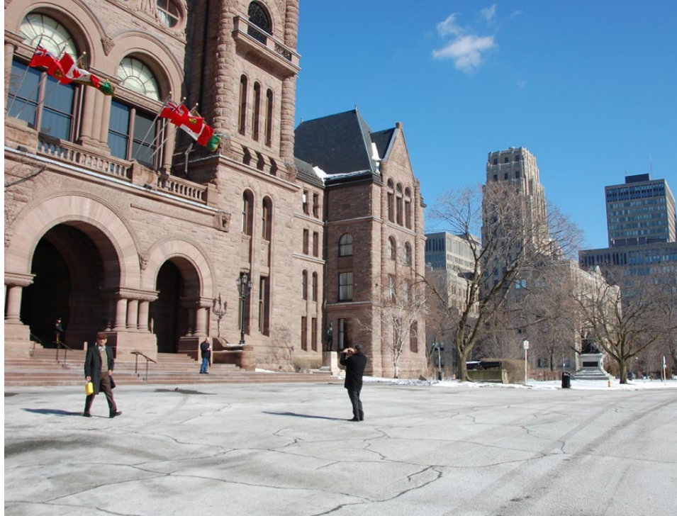
Fig 2.51: Run down road at Entry
