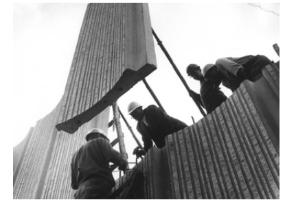
Fig 2.25: Lifting in the concrete panels with vertical fluting.
