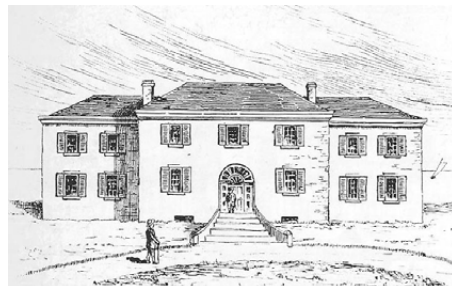
Fig 2.35: Parliament Buildings erected in 1820, burned down in 1824
