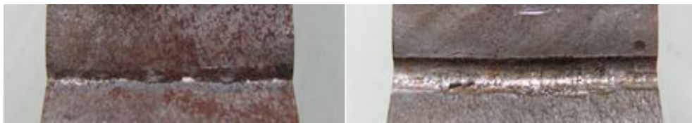
Figure 3.5: Weld toe of A1 (left) and F6 (right)
