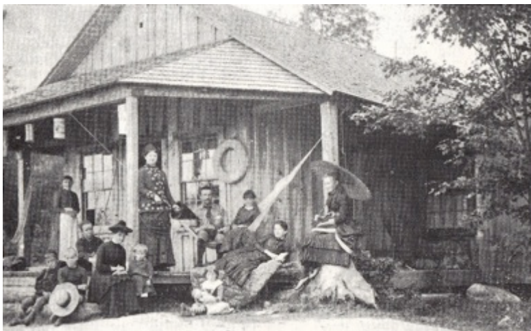
Figure 4:7. James Campbell's Cottage, Lake Joseph, 1886. Source: Mason, First Islanders , 1974.
