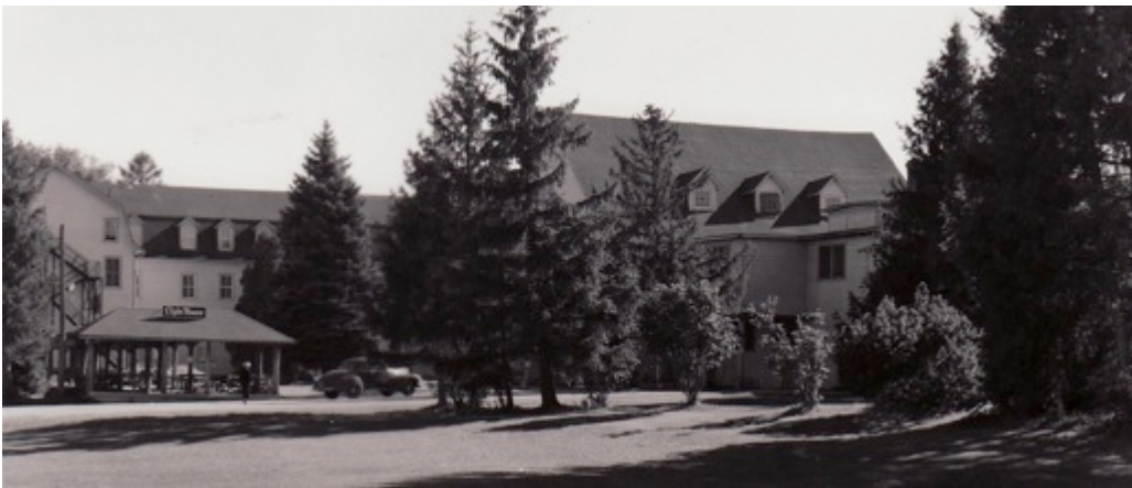
Figure 4:82. Motor Entrance, Elgin House, c1940. Source: Muskoka Boat and Heritage Centre.
