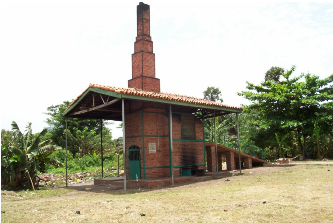
Figure 7.11: Mass Burn Incinerator at a Healthcare Facility in Accra. Photo by Squire, 2010
