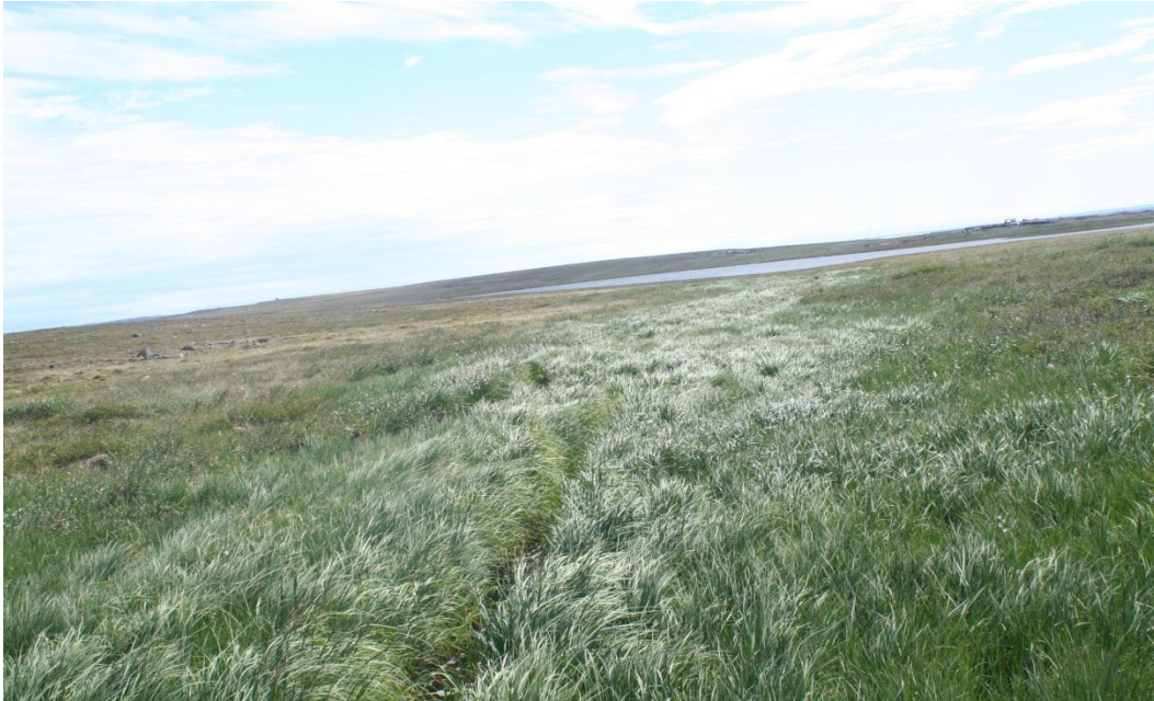
Figure 38. Baker Lake tundra municipal wastewater treatment wetland.
