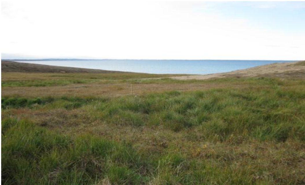
Figure 42. Paulatuk tundra municipal wastewater treatment wetland.
