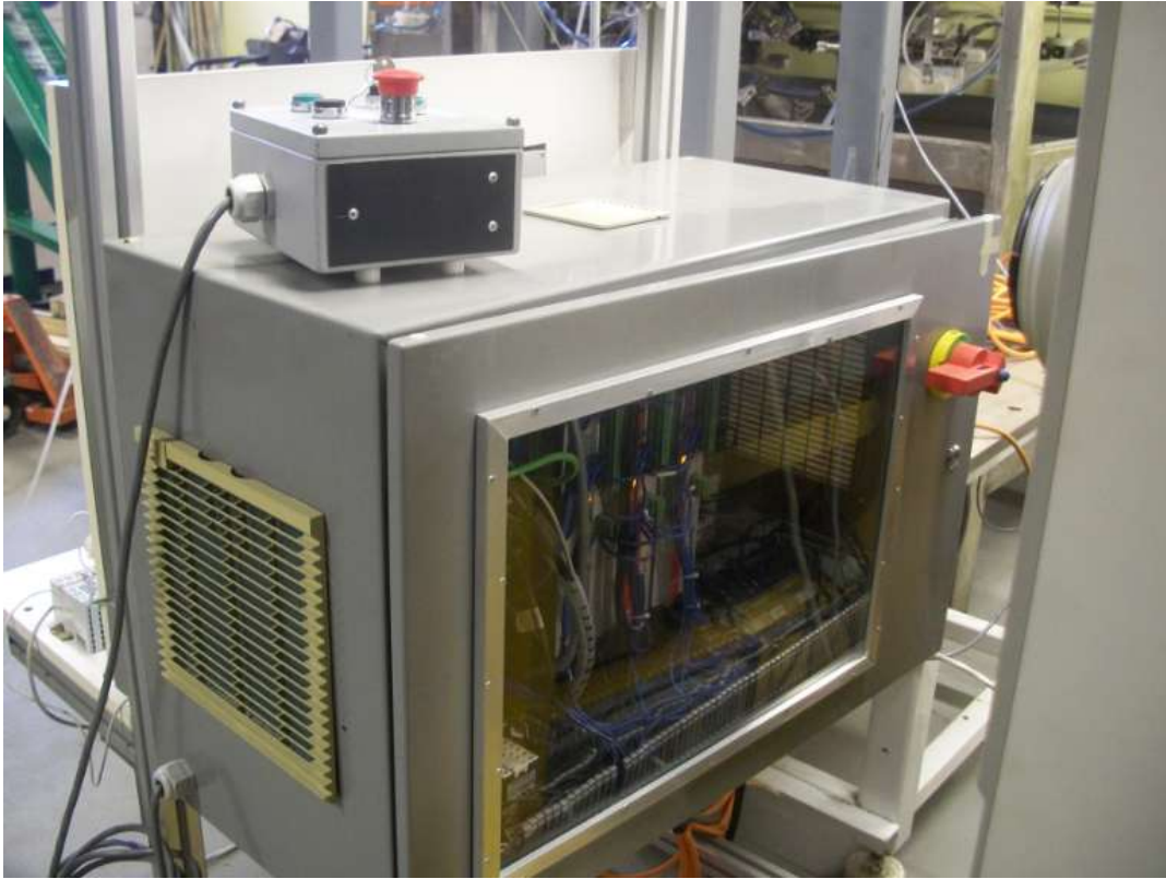
Figure 7-5: Photograph of the Control Box
