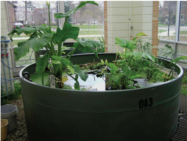
Fig 2.36 Typical cell of a Living Machine®
