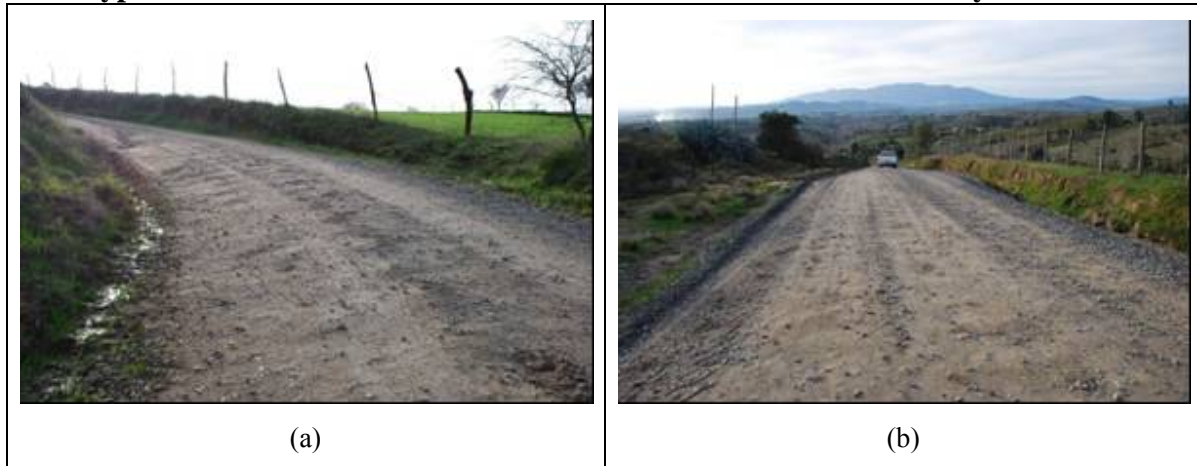
Figure E.1.1 Corrugations in Roads (a) N462 and (b) N480
