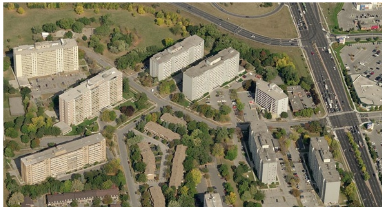
Fig. 3.4 The tower in the park model is an early high density residential typology used extensively in Toronto's suburbs
