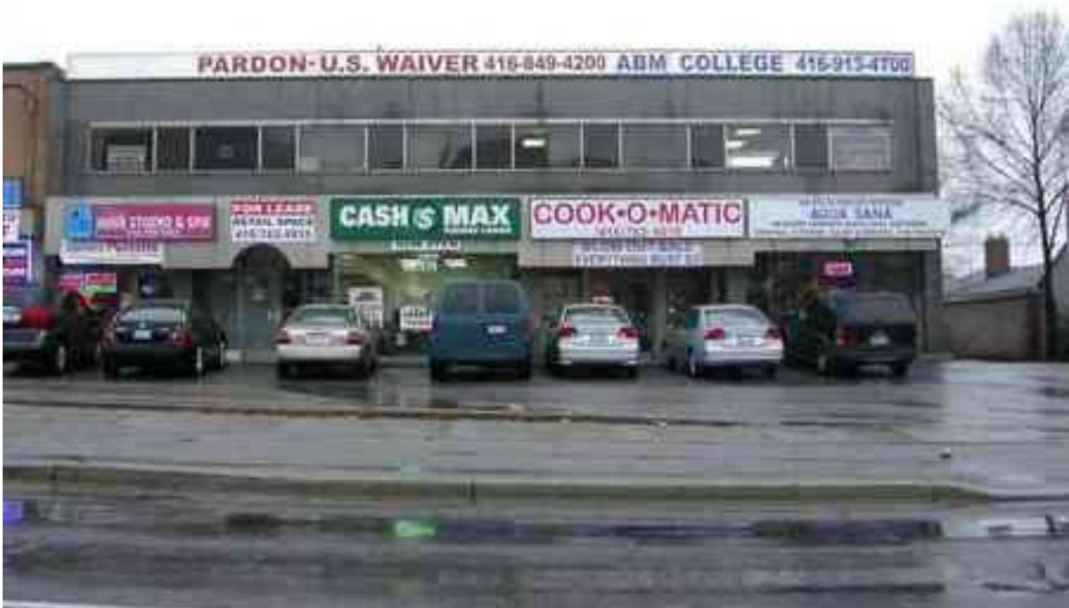
Fig. 1.12 A typical suburban strip mall is designed for use by drivers primarily
