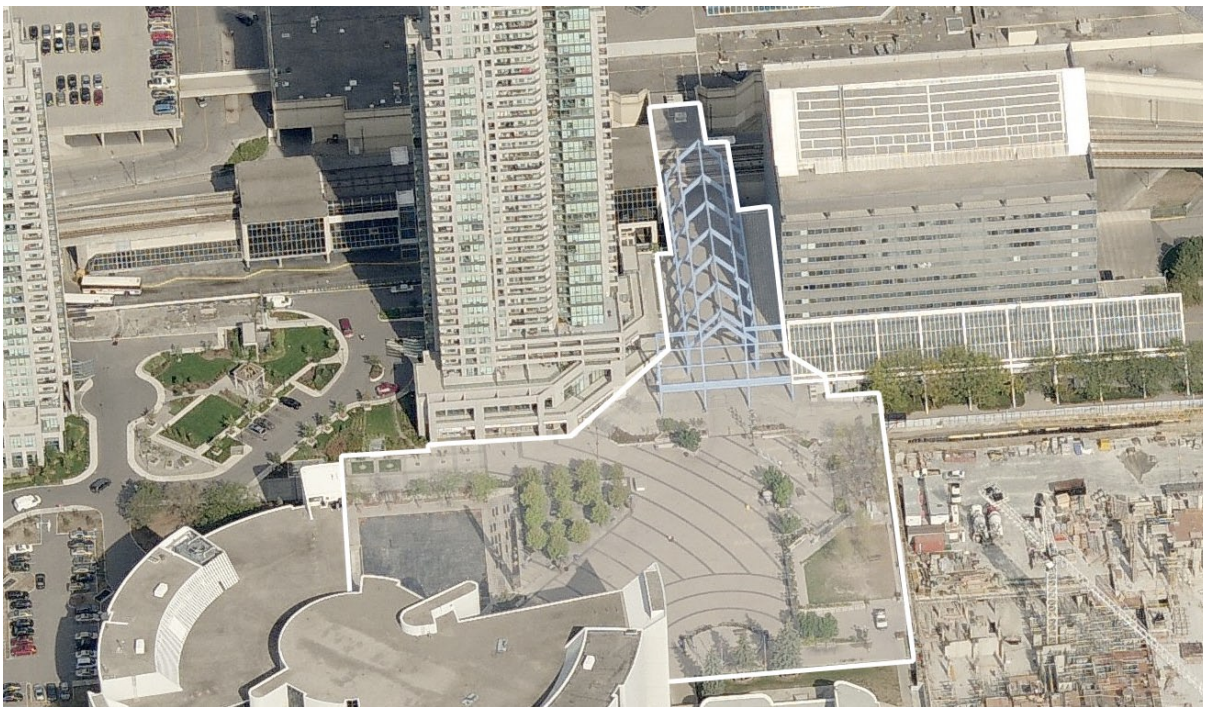
Fig. 4.10 Albert Campbell Square connects to a pedestrian bridge up to the SRT station entrance and the upper level of the mall
