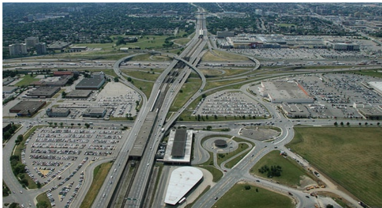
Fig. 2.1 Extensive parking lots and regional bus stations at Yorkdale and Wilson Stations collect suburban commuters
