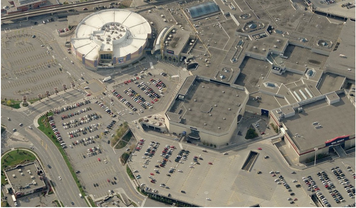
Fig. 4.9 Extensive surface parking lots and decks surround the mall on three sides
