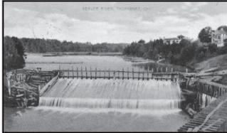
◀ Thornbury's first dam was a primitive one, built in the 1850s when the town was settled. It was constructed to supply power supply to the adjacent mill.
