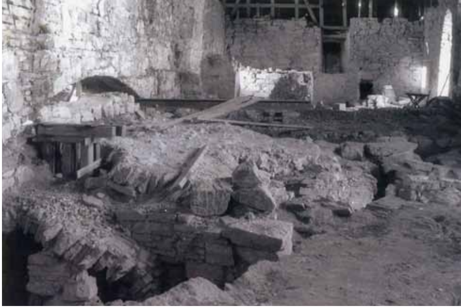
6.43 State of barn before the renovation
