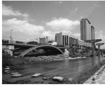
Fig.3.27 Freeway support's remain to symbolize the river's history.
