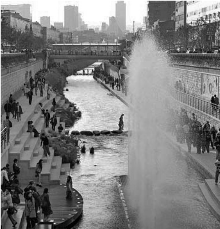
Fig.3.24 The city removed an elevated highway and restored a river into a public parkway.
