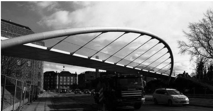
Fig.2.44 Bicycle and pedestrian bridge.
