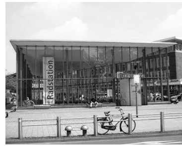
Fig.2.48 Elevation of the main entrance to the Radstation.
