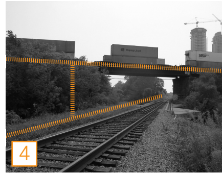
Fig.4.12 Junction Box - Medium (raised intersection of rail corridors)
