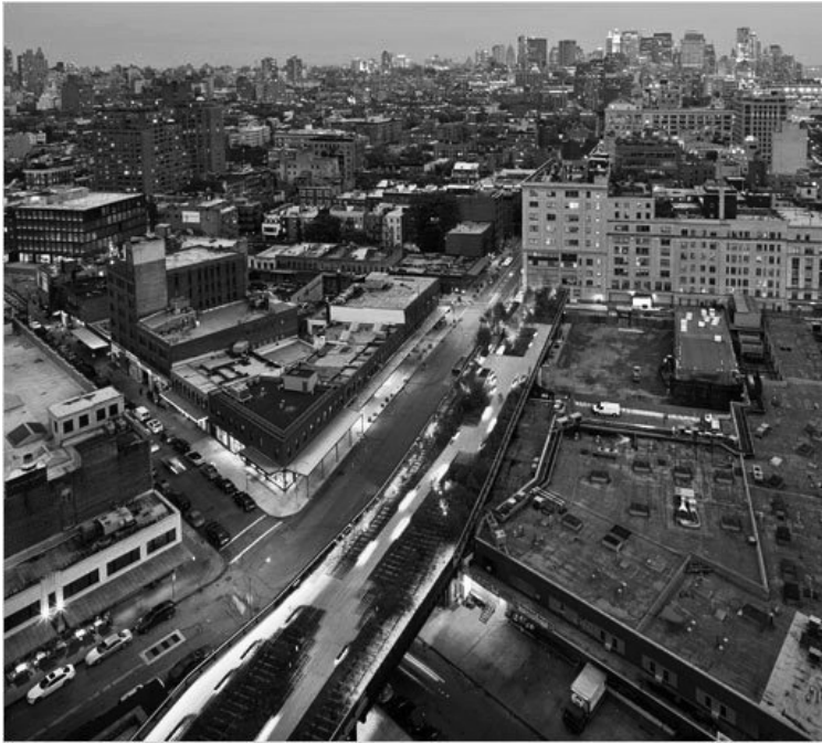
Fig.3.13 Section one completed, Gansevoort Street to 13th Street, view looking south from the Standard Hotel.
