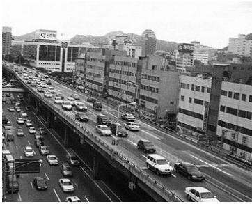
Fig.3.26 Cheonggye elevated free-way separated Seoul's city centre.
