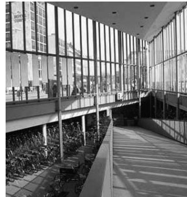
Fig.2.50 Interior of the Radstation.
