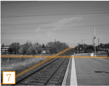
Fig.4.6 Junction Box - Heavy (intersection of a hydro and rail corridors with a transit station)
