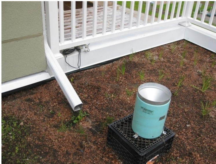
Figure 5: Downspout connecting the Archetype House roof to the greenroof.
