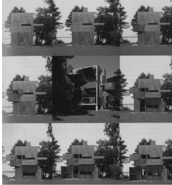
A 4m x 6m x 7m wooden frame with moveable walls that can be manipulated by the occupant, transforming this experimental house from a static object to a sequence of experiences.
