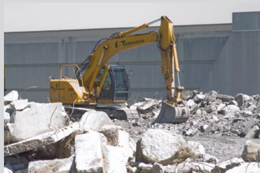
fig. 1.01: Demolition site of Constellation Hotel, Etobicoke, ON. Photo by author, 2008.
