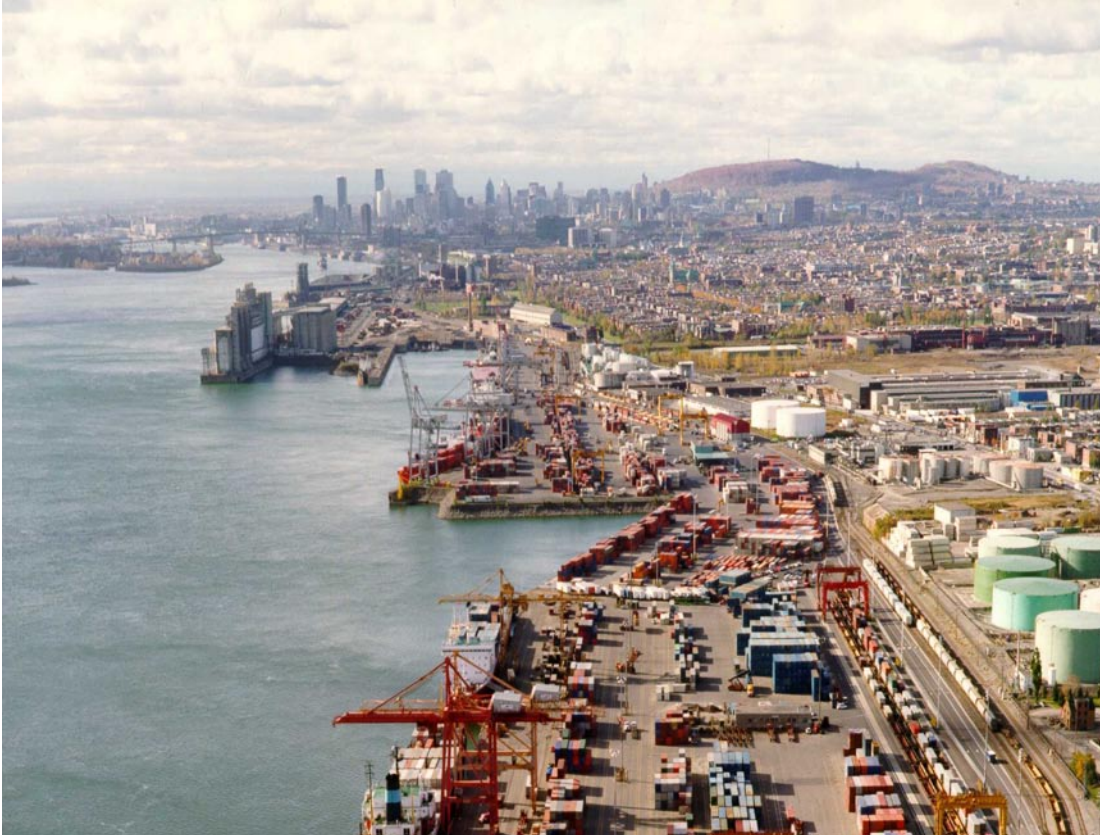
fig. 1.02: Aerial view of Montréal's Modern Port Facilities. Courtesy Port of Montréal, 2006.
