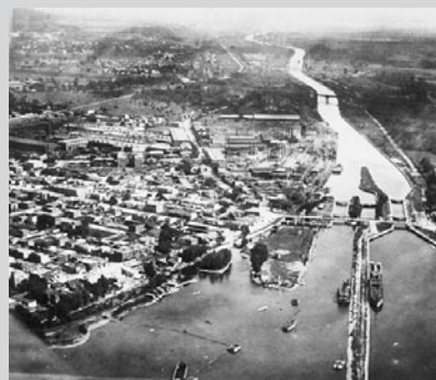
fig. 3.01: Lachine Canal inlet facing northeast, Lachine, QC. Courtesy Parks Canada, c.1920.
