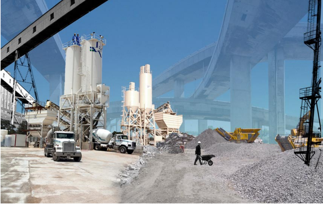
fig.4.04: Envisioning temporary concrete production at Turcot. Photomontage by author, 2008.
