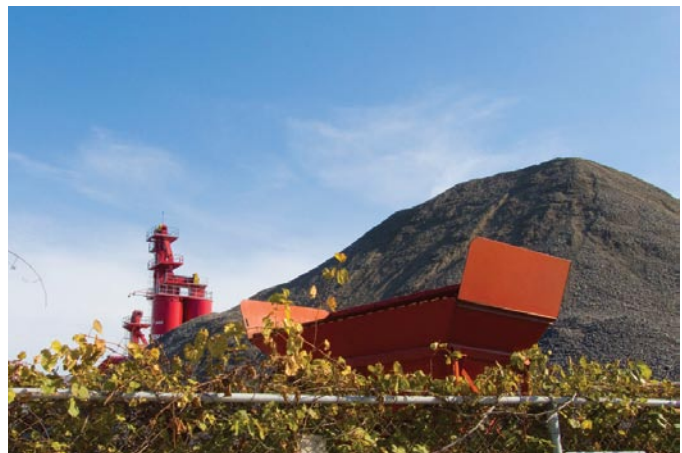
fig. 2.06: Aggregate stockpile at Construction DJL, Lachine-Turcot District. Photo by author, 2009.
