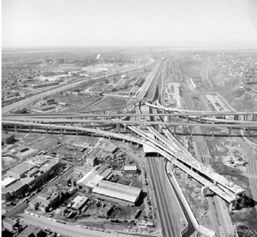
figs. 3.22–3.24: Views of Turcot Interchange nearing completion, c.1967. Credit: Gabor Szilazi, courtesy BANQ.
