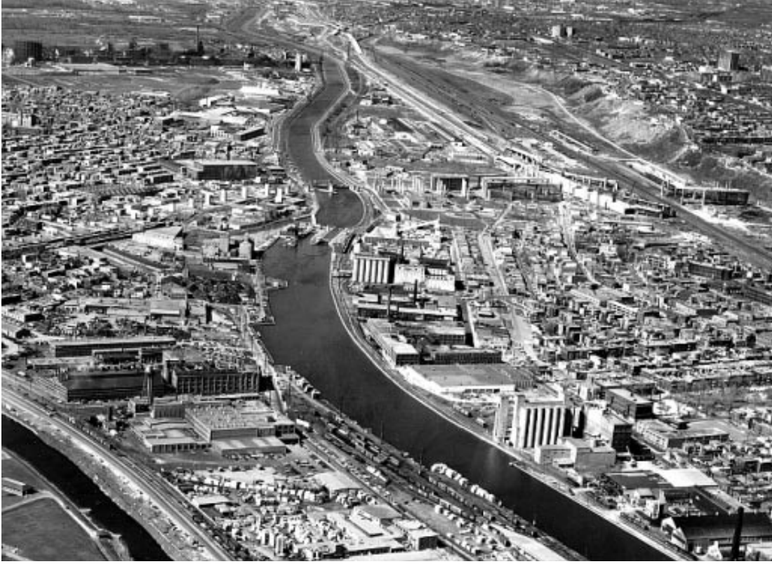
fig.3.25: Aerial view of Turcot-Lachine District showing granaries in foreground, autoroute construction midground, and LaSalle Coke operations in background. c.1965. Credit: Gabor Szilasi, BANQ.
