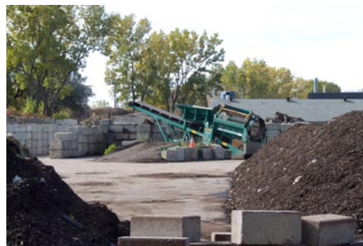
fig.2.04, bottom: Holcim Concrete Plant, Lachine-Turcot District. Photo by author, 2009.
