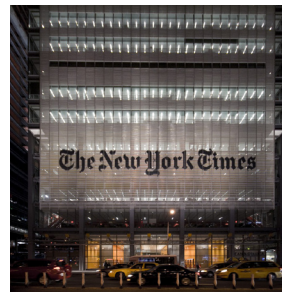
Fig 5.15 New York Time Building, day and night views Renzo Piano Building Workshop
