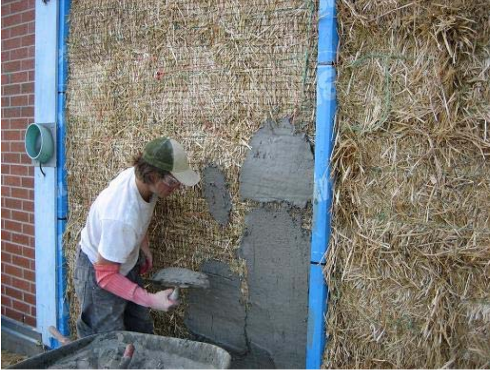
Figure 41. Applying the cement plaster.
