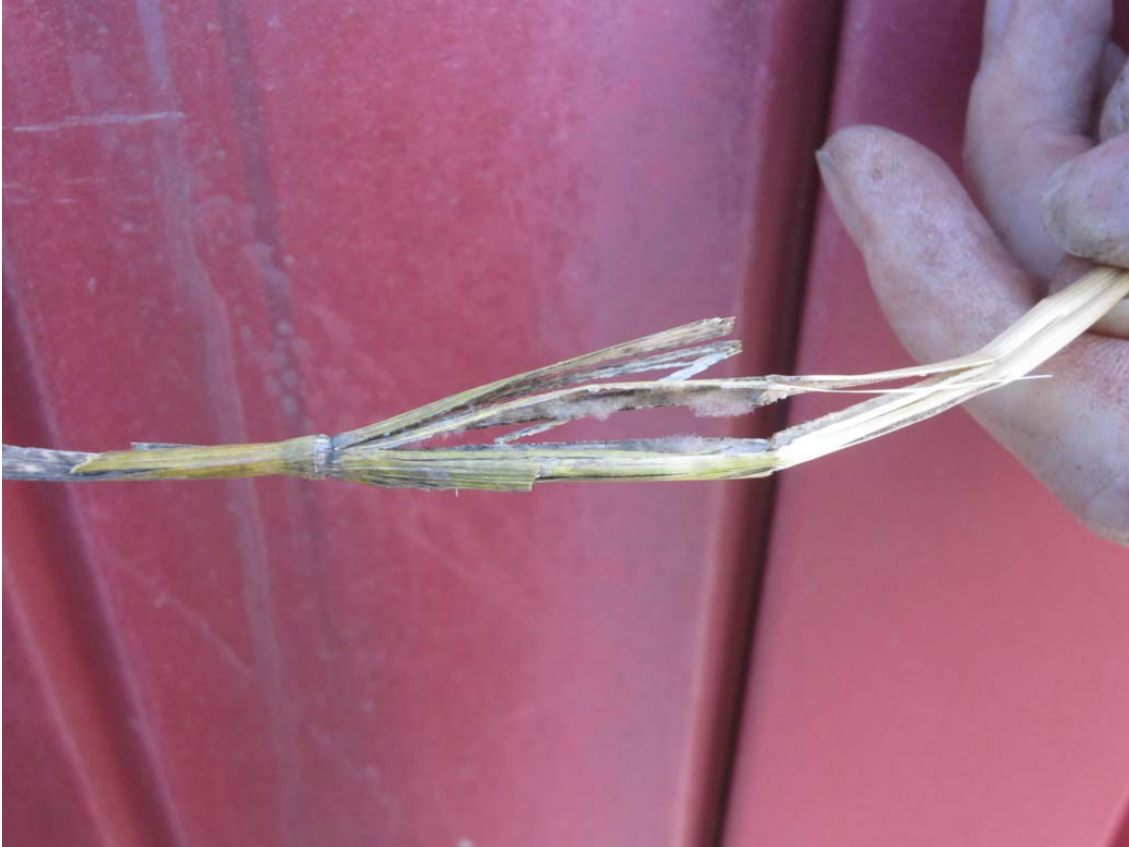
Figure 81. Photograph of the highest level of mould growth in the clay plaster wall.
