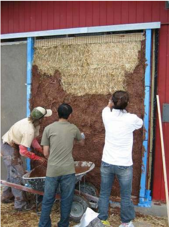
Figure 42. Applying the clay slip.
