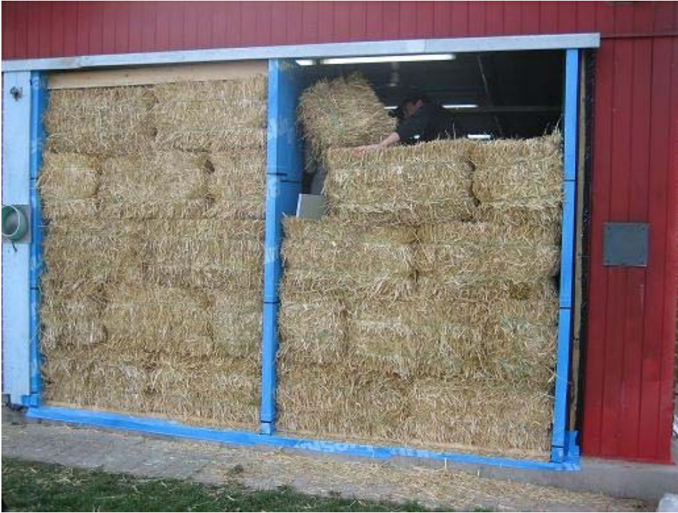
Figure 40. Stacking the straw bales for the test walls.
