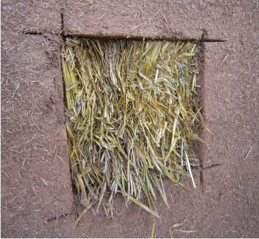
Figure 79. Clay plaster removal (12"x12") exposing straw behind.
