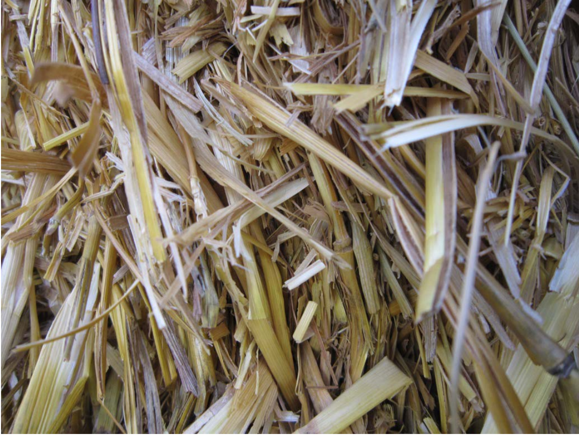
Figure 80. Photograph showing the straw behind the clay plaster.
