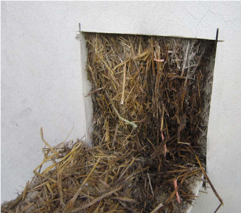
Figure 78. Cement plaster removal (12"x12") exposing straw behind.
