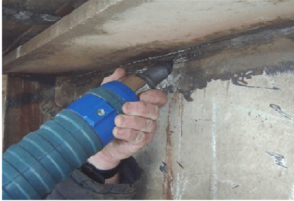
Figure 1.1: View of the zone of repair (welding +UP treatment) of fatigue crack in welded element of bridge span (left) [Kudryavtsev et al. 2005], and needle peening a weld toe in [Walbridge 2005] (right)
