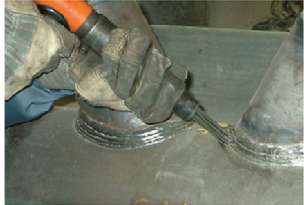
Figure 1.1: View of the zone of repair (welding +UP treatment) of fatigue crack in welded element of bridge span (left) [Kudryavtsev et al. 2005], and needle peening a weld toe in [Walbridge 2005] (right)
