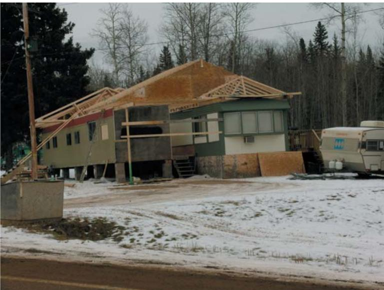
groundplane collapse and/or the slow subsistence of the building into the earth. In either case, differential settlement – whether slight or extreme – can cause havoc to a building's structure..
